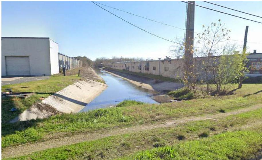
The concrete-lined channel drains east and merges into E101-18-00 where it crosses I-45 at Outfall C4. The existing drainage layout is shown in **Exhibit 4**, and the existing offsite drainage layout is shown in **Exhibit 5**. Outfall O7 meets the main lane and frontage road drainage design criteria as shown in **Table 2**.
