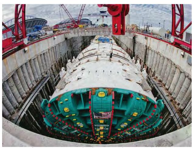
**Figure 3.** Large diameter EPB-TBM prior to launch at SR-99 tunnel project in Seattle, WA (Source: Tunnel Business Magazine, August 2013 ed., p.28).
