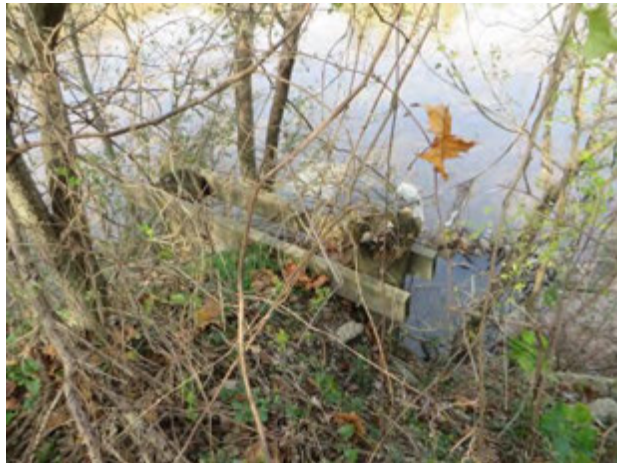
Figure 34. Scaffold and drainage pipe into Buffalo Bayou, southern bank, looking north
