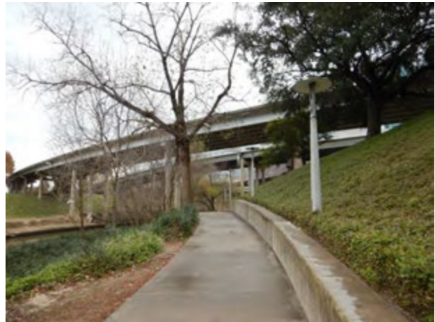
Figure 54. Looking east towards APE along Buffalo Bayou. Note lights along path.
