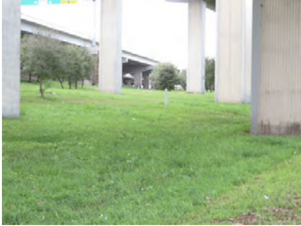
Figure 26. Looking South down the APE along US 59. Note the berm sloping away from the main lanes.
