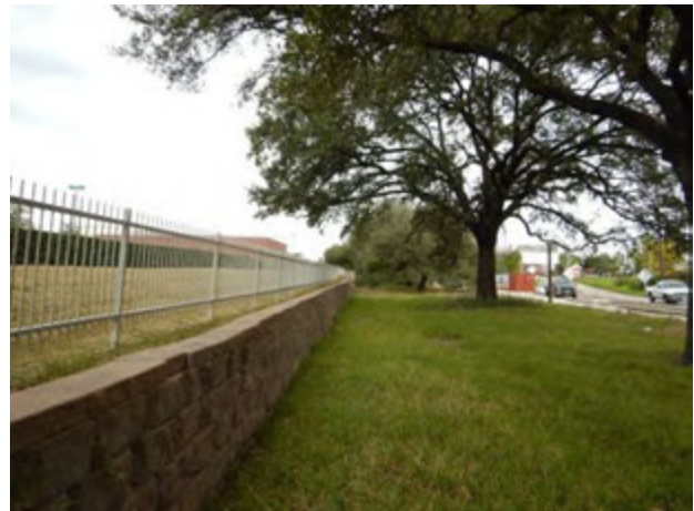
Figure 44. Looking north along Parcels No. 54 and No. 55.
