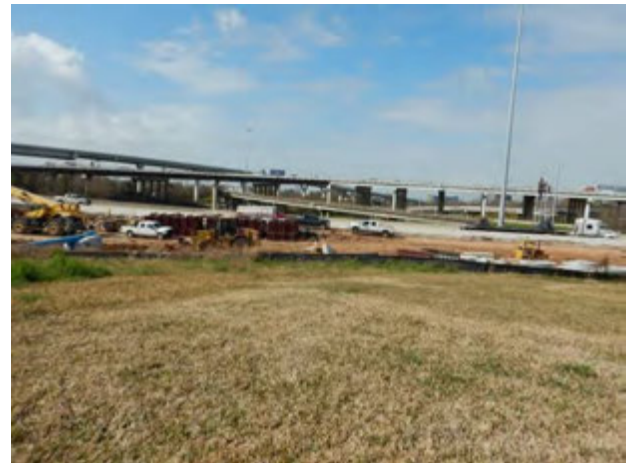
Figure 36. Looking west towards highway construction near Shovel Test No. 32.
