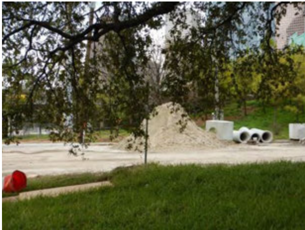
Figure 47. Highway construction at Allen Parkway and Heiner Street.
