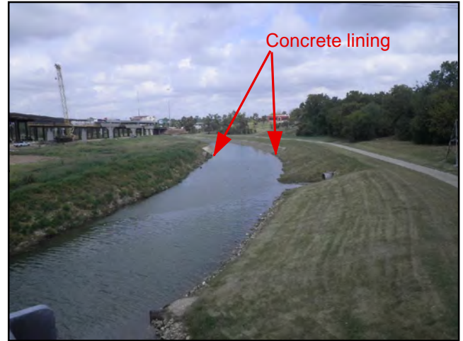
Photo 22 - Looking north from bicycle path bridge at White Oak Bayou (riprap-lined banks in foreground to concrete-lined banks in background)
