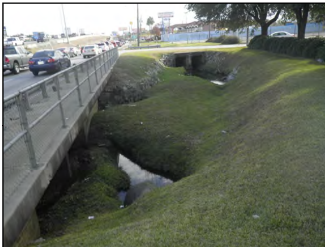
Photo 10 - Looking south at Wetland 4 (culverts and sediment deposits in channel)
