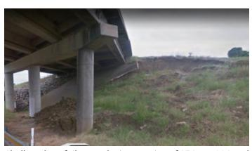
Shallow slope failure at the intersection of SE Loop 286 and Clarksville Street, Paris, Texas.
