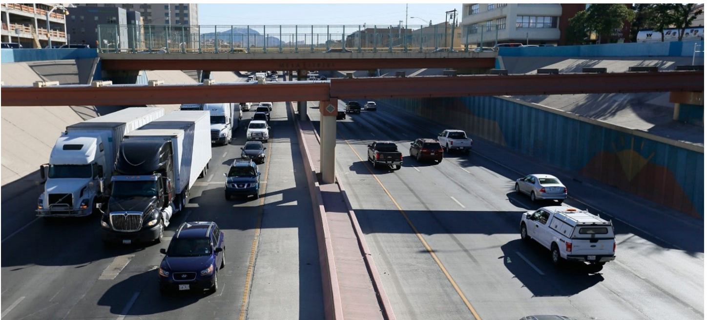
Figure 4: Existing Westbound View at Mesa Street
