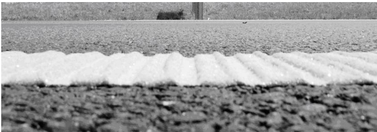
Figure 2-12. Typical inverted-profile thermoplastic marking (profile view).
