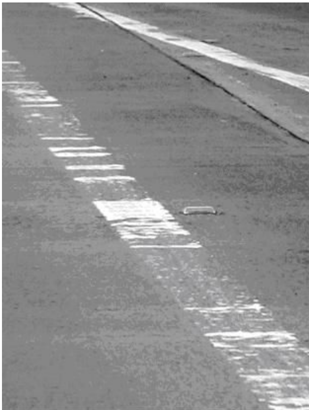
Figure 2-11. Major thermoplastic failure on concrete.
