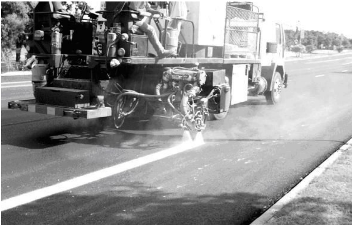
Figure 2-10. Typical sprayed thermoplastic operation.
