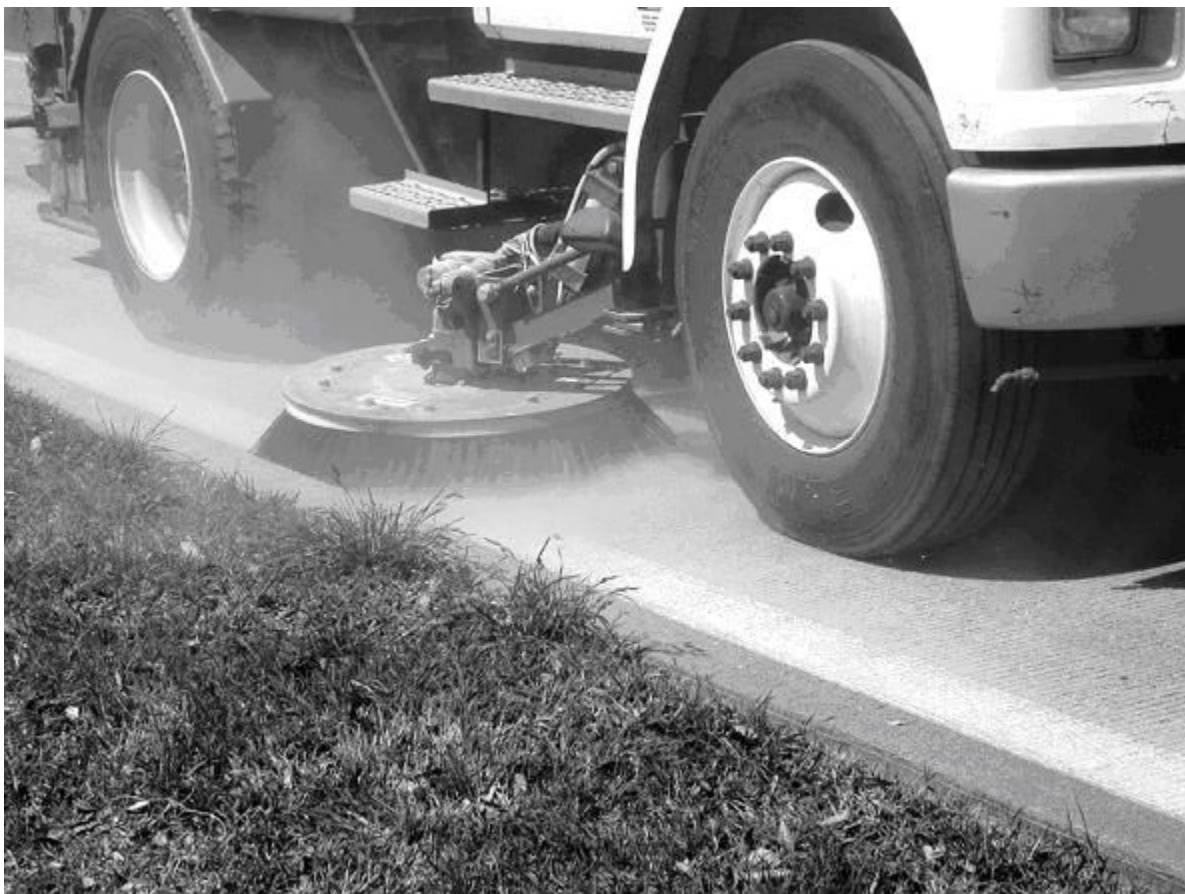
Figure 2-8. Typical brooming operation for surface cleaning prior to striping.
