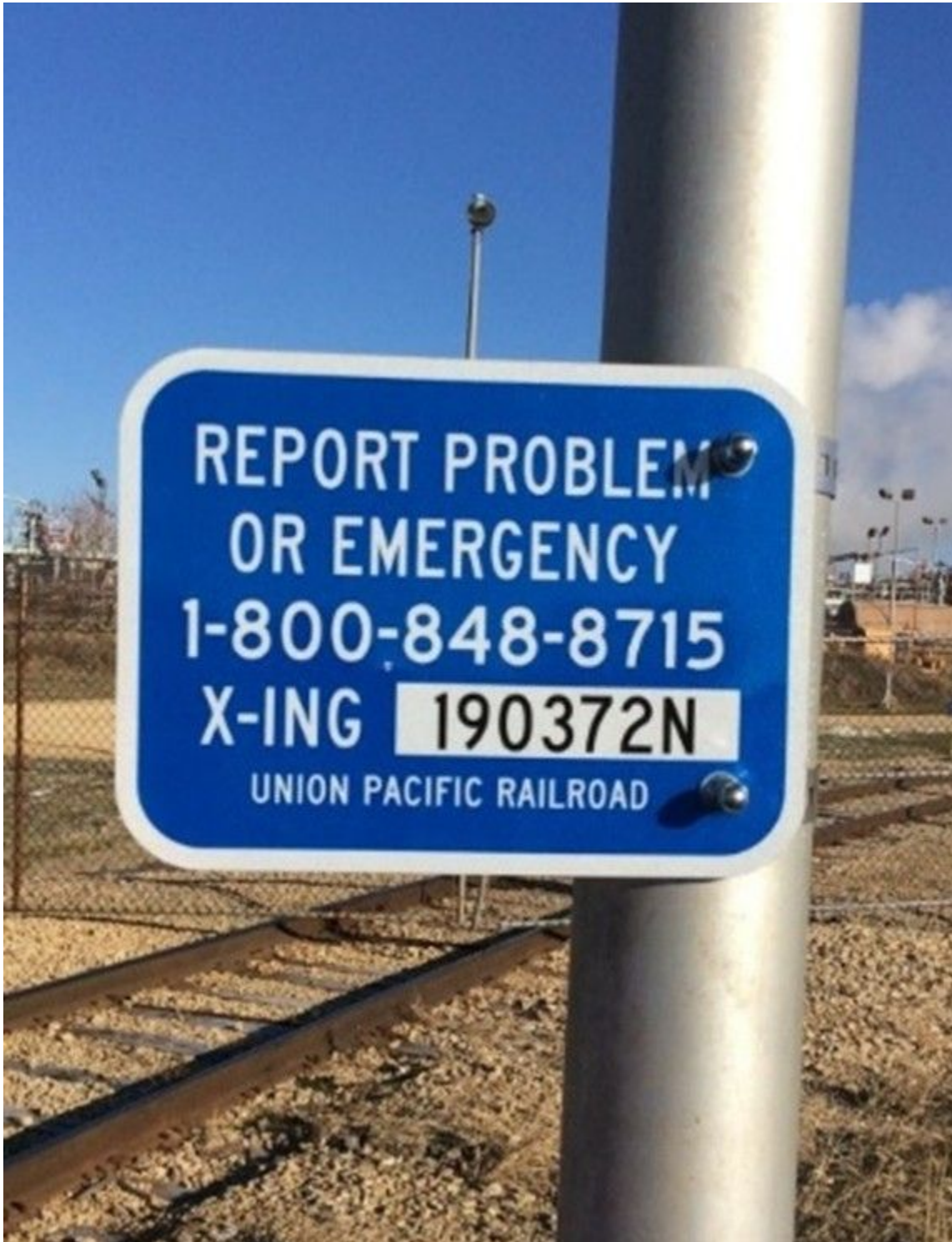
Figure 8–1. Emergency Notification System (ENS) sign
