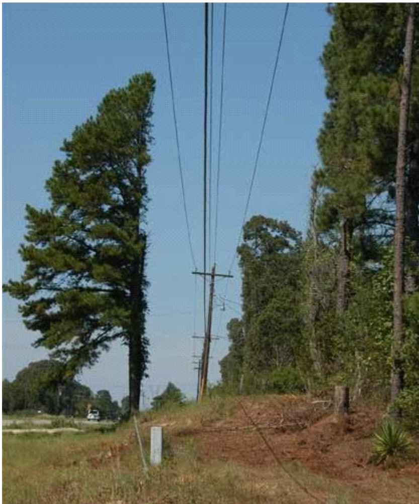
Figure 4-20. Unbalanced, unsafe and unsightly tree pruning by utility company. Trees should have been removed by utility company for safety and aesthetic reasons.
