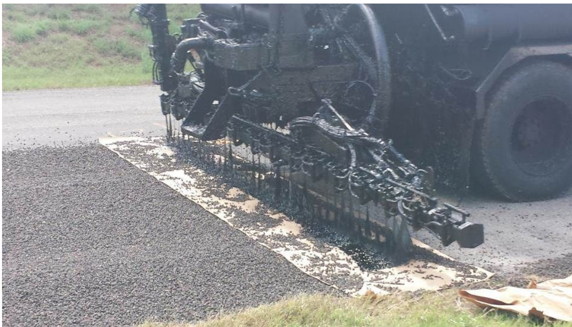
Figure 8-6. Correct Starting Position over Paper Joint.
