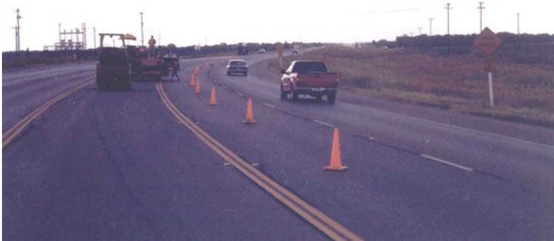
Figure 8-1. Traffic Cones in Position.
