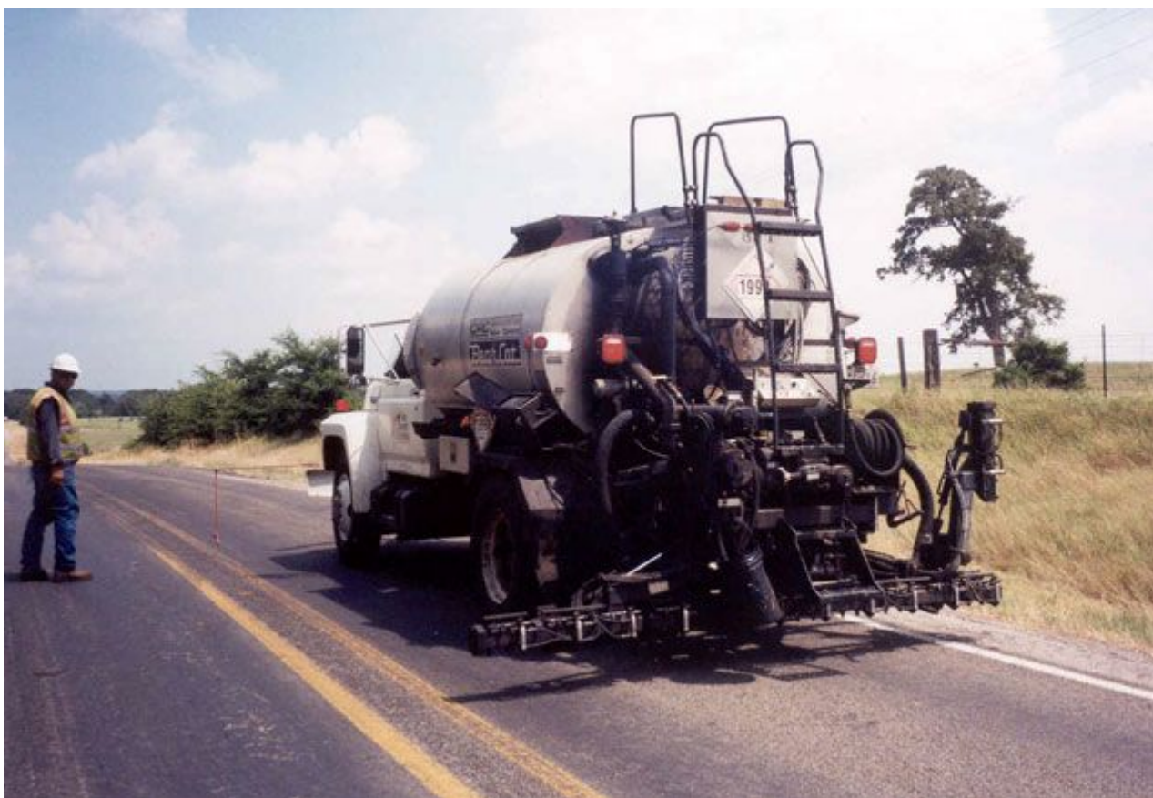
Figure 7-11. Typical Distributor Spray Bar.
