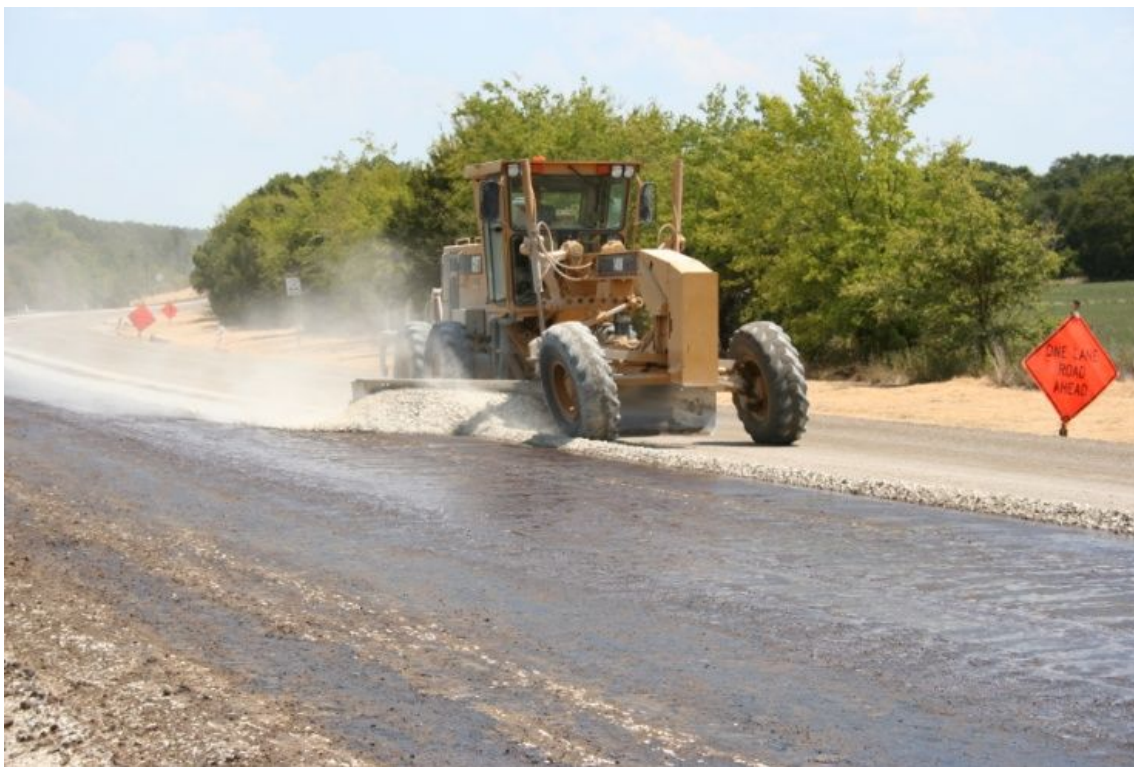
Figure 1-6. Worked-in (cut-in) prime.
