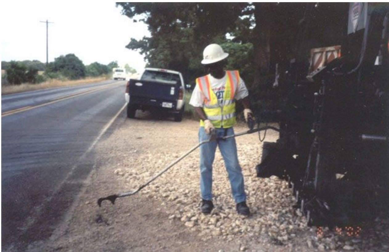
Figure 7-22. Typical Hand Sprayer on Asphalt Distributor.
