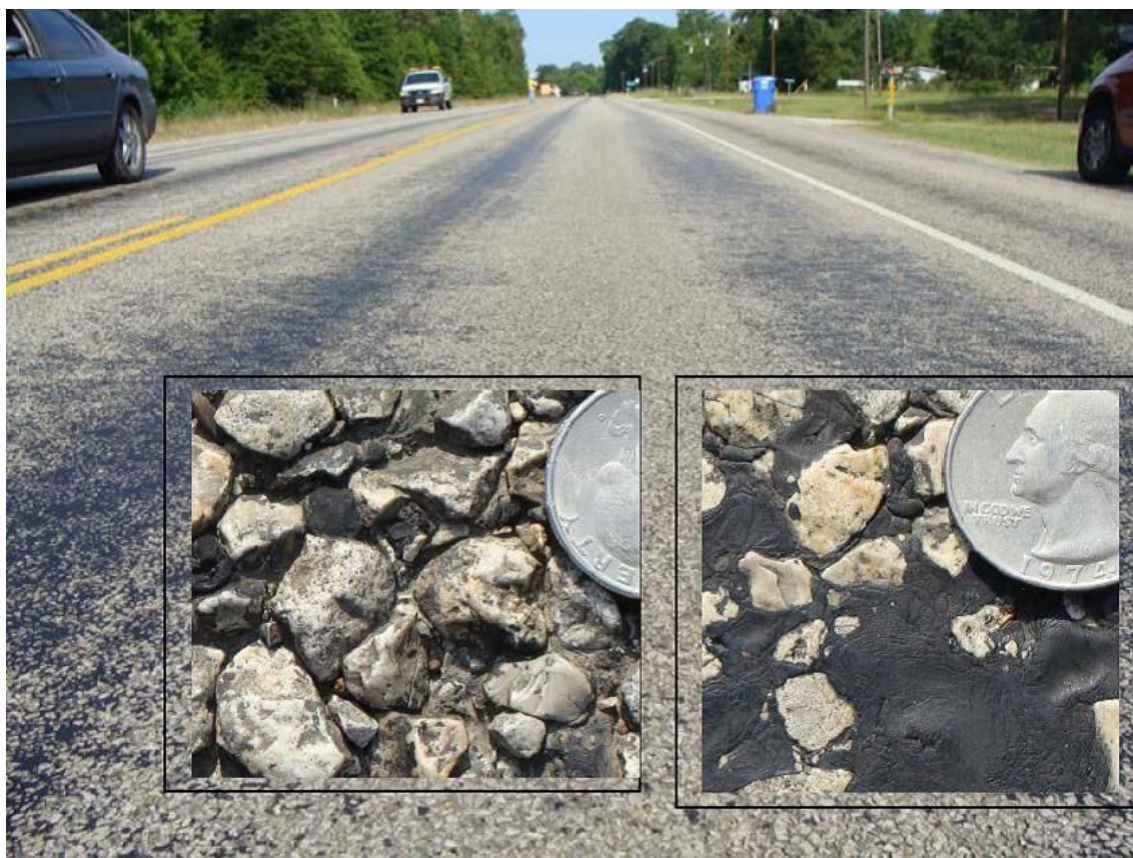
Figure 4-2. Pavement texture varying across a pavement.
