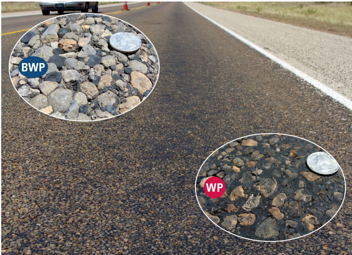
Figure 4-5. Lane with moderate flushing.
