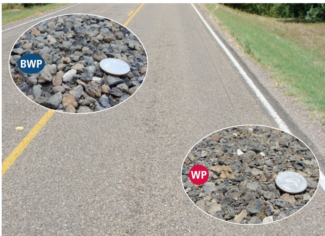
Figure 4-8. Lane with slight wheel path color difference.
