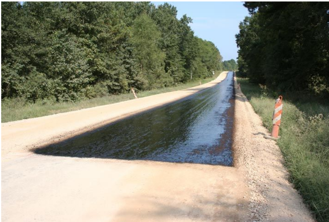
Figure 1-5. Spray-applied prime (MC-30 or AEP).
