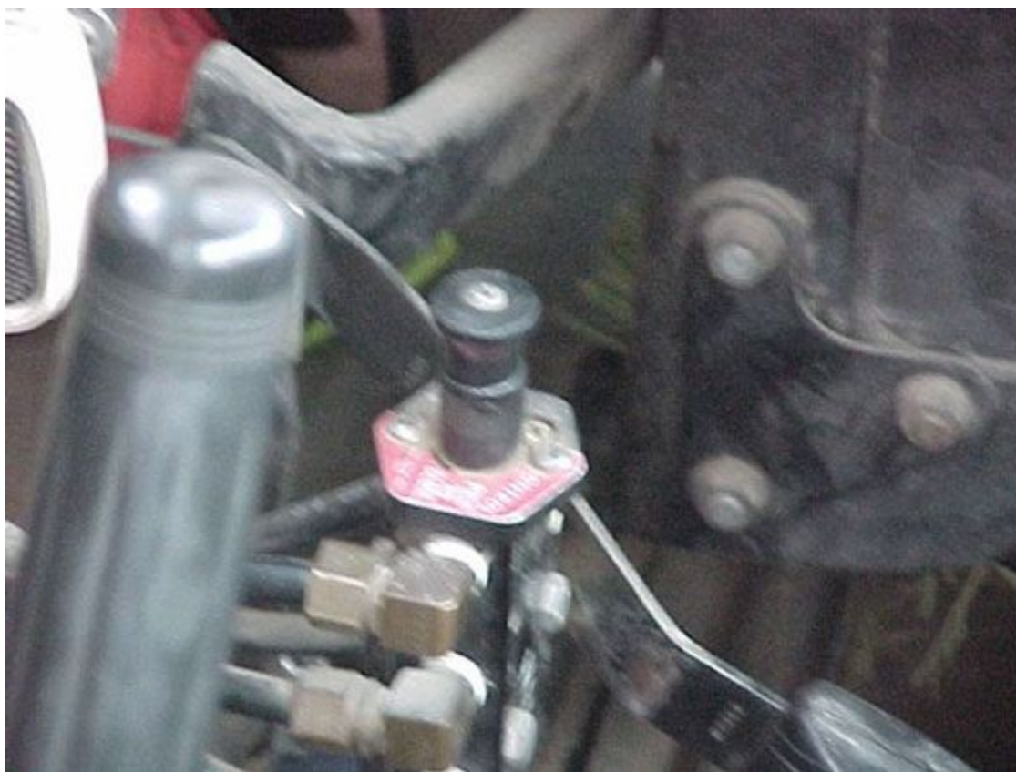
Figure 7-35. Control Valve in Truck Cab.
