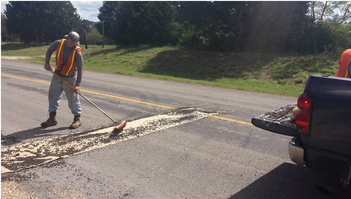
Figure 8-3. Placing a Paper Joint at Beginning of Shot.
