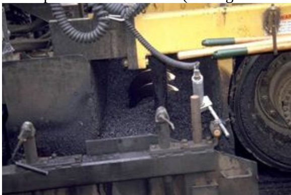
Figure 6-29. Augers distributing HMA. © Copyright 2006 University of Washington
