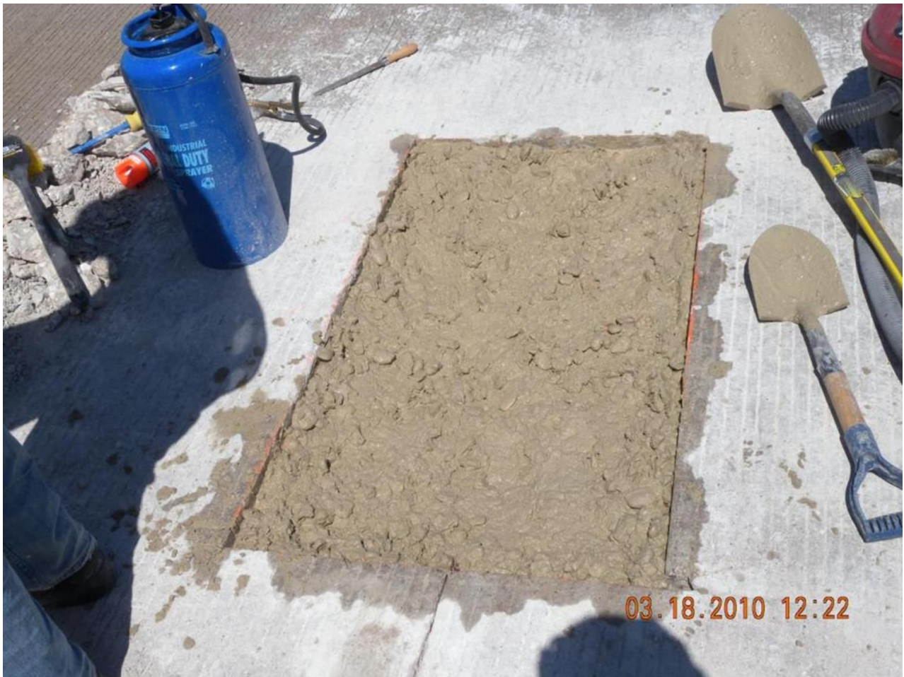
Figure 10-12. Place repair materials.
