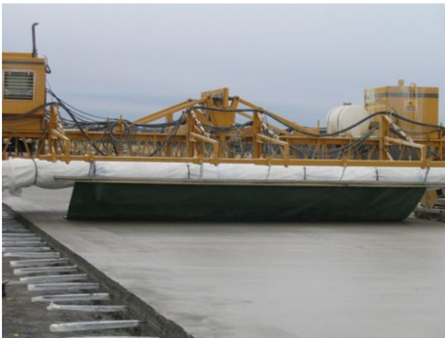
Figure 9-60. Mounting of artificial carpet.
