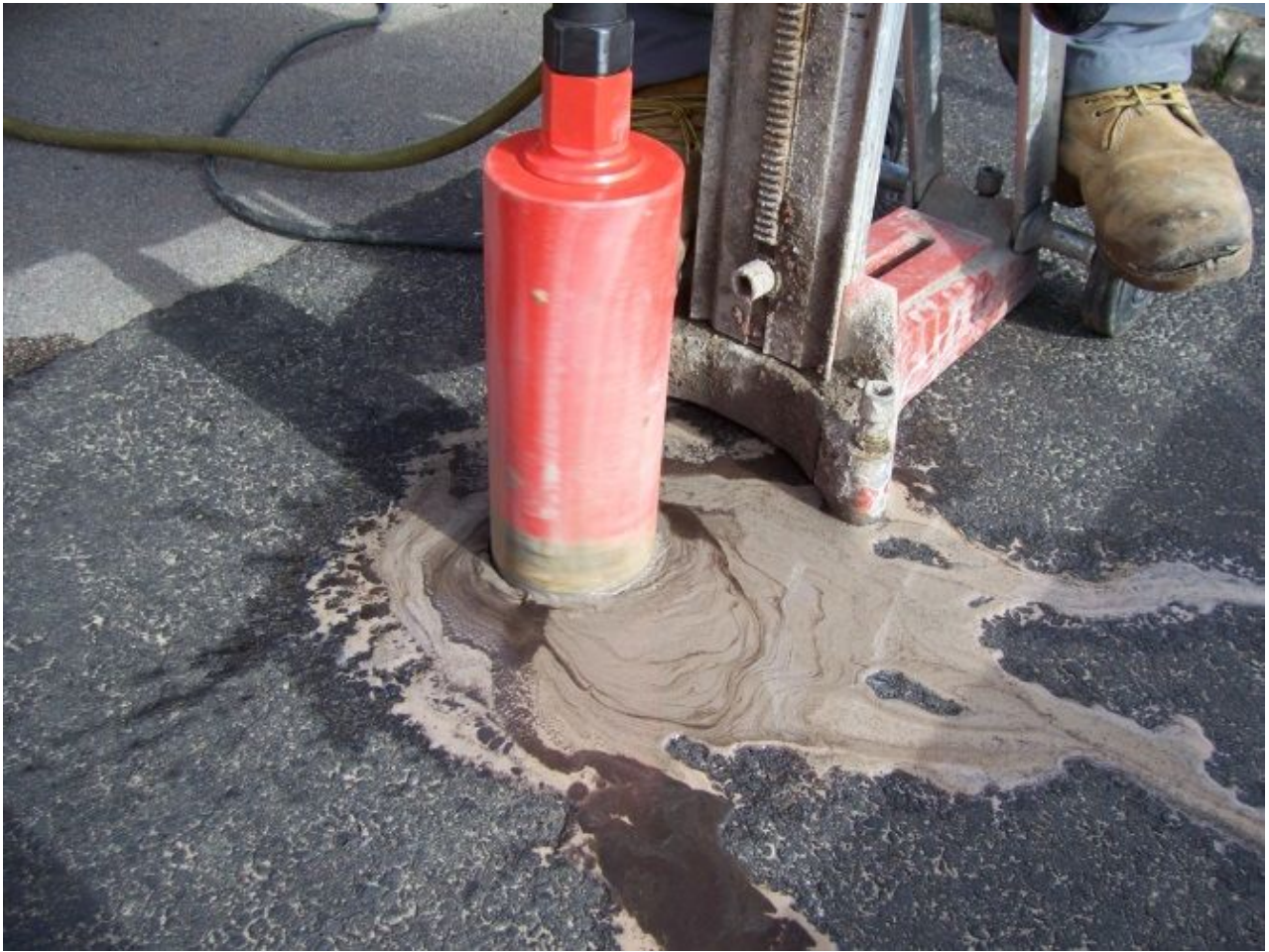
Figure 6-52. Core extraction. © Copyright 2006 University of Washington
