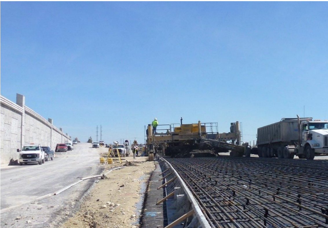
Figure 9-24. Side forms used for paving.
