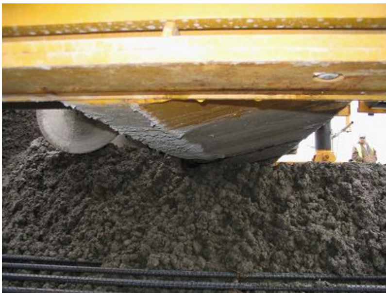
Figure 9-43. Auger and strike-off spreading the concrete.
