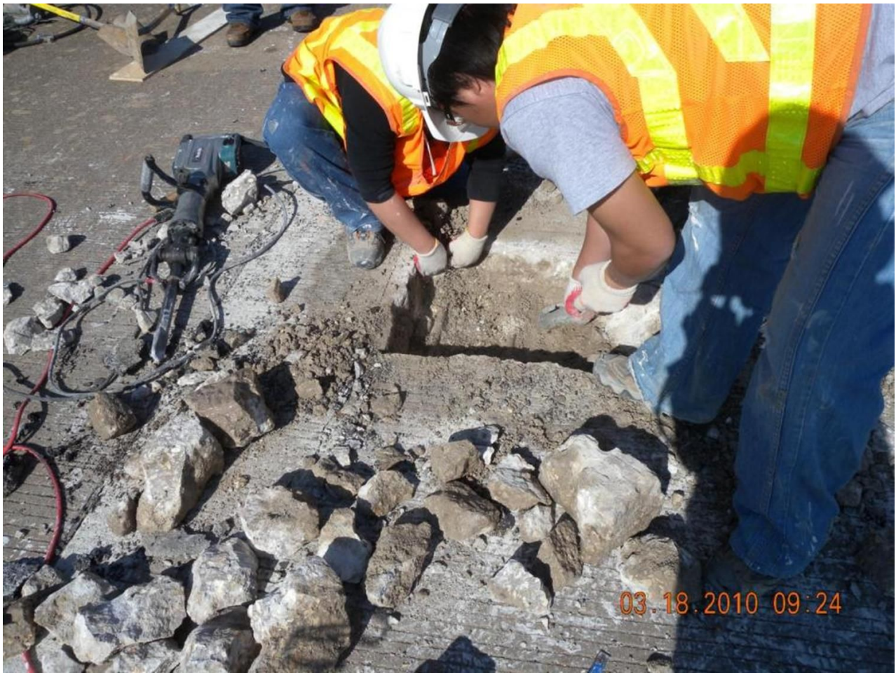
Figure 10-10. Removing deteriorated concrete.
