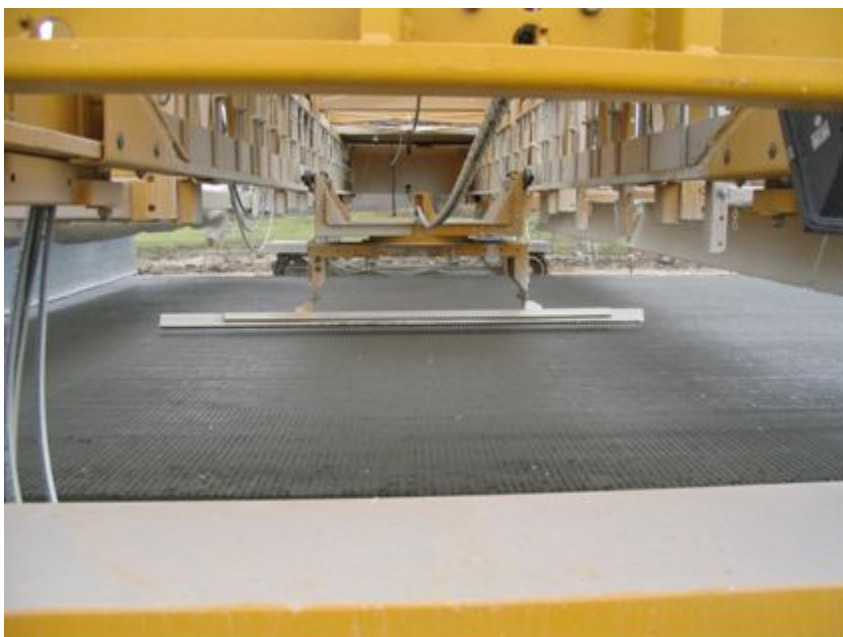
Figure 9-62. Mechanical tining device.
