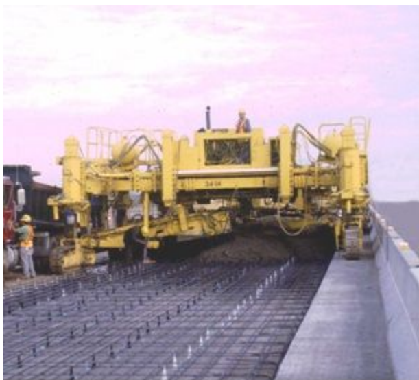
Figure 9-33. Paver machine on tracks.
