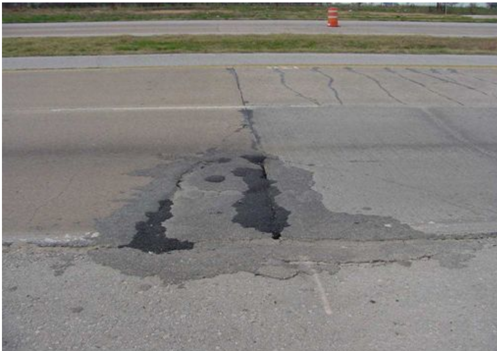
Figure 10-3. Full depth repair of punchouts in CRCP.
