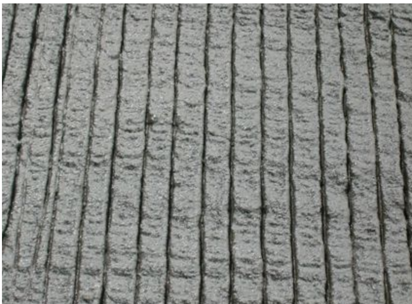
Figure 9-61. Transverse tined Surface.
