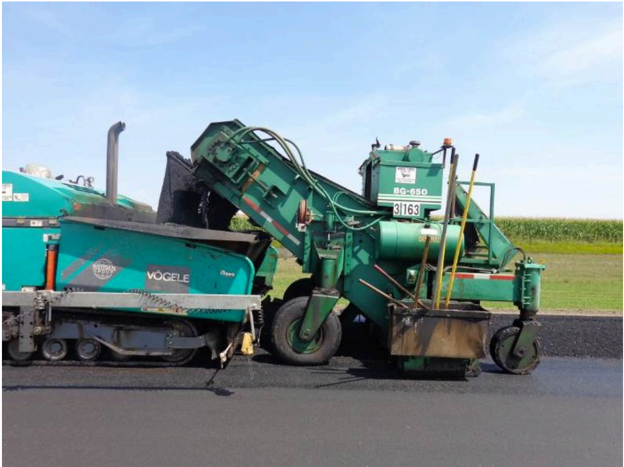
Figure 6-45. Windrow paving. © Copyright 2006 University of Washington
