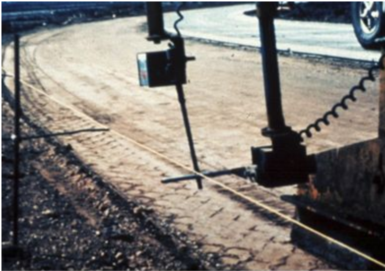
Figure 9-37. Horizontal and vertical sensors.
