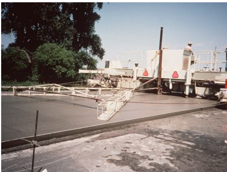
Figure 9-52. "V" shaped drag float pulled by paver.
