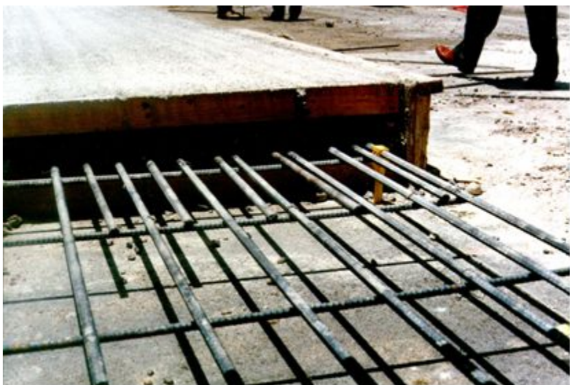
Figure 9-76. Additional steel is required at header.
