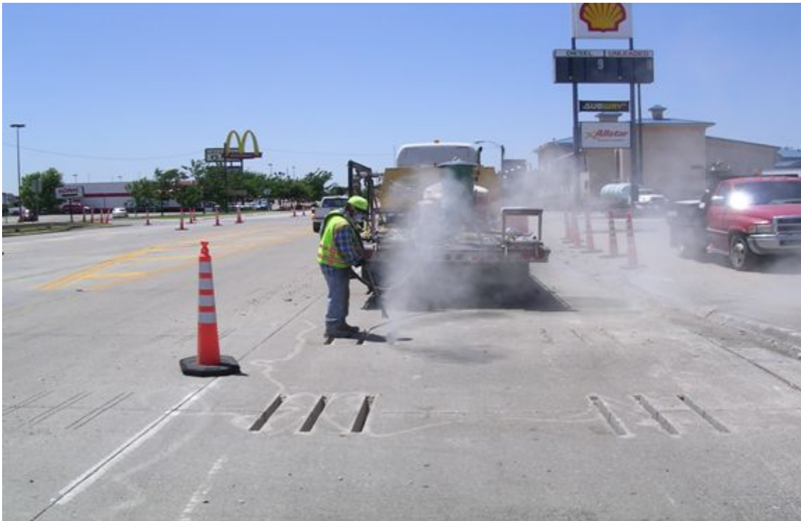
Figure 10-21. Sandblasting the slots.
