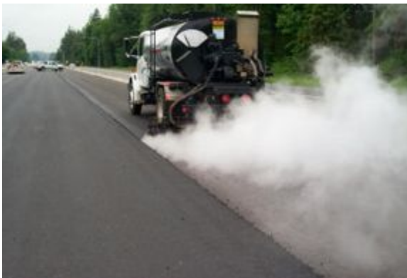
Figure 6-9. Tack coat application. © Copyright 2006 University of Washington
