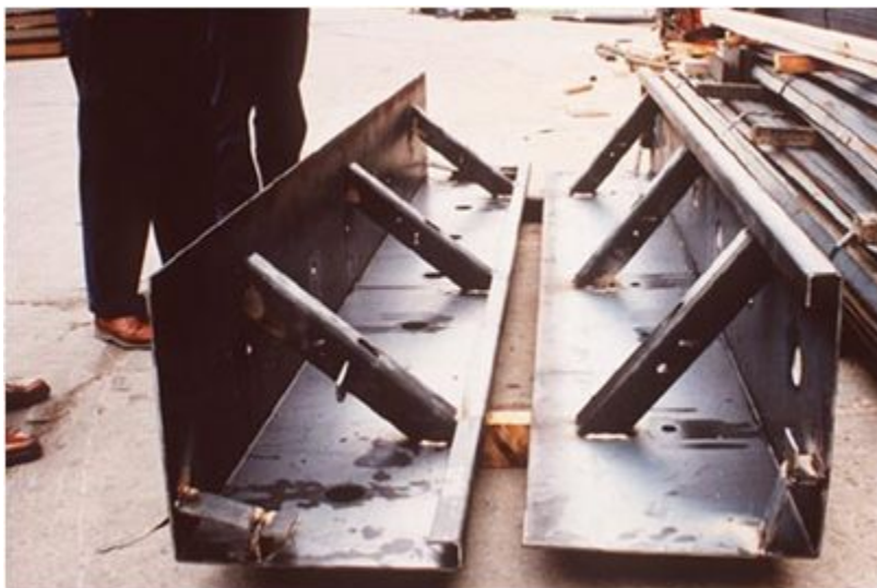
Figure 9-21. Forms ready for setting.
