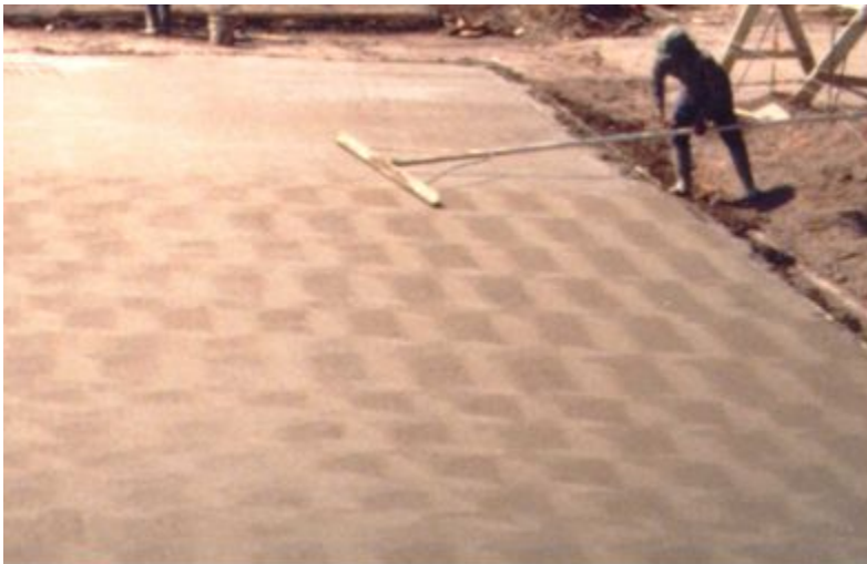
Figure 9-56. Straightedge finishing behind a longitudinal float.
