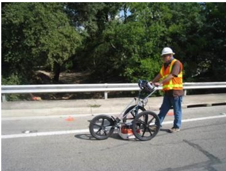
Figure 4-11. 400 MHz Ground-coupled Penetrating Radar.
