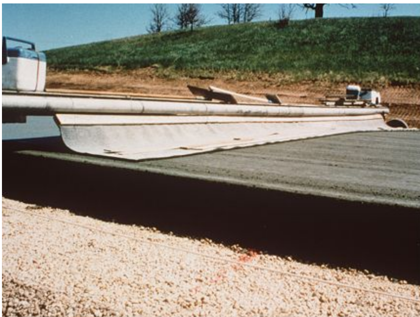
Figure 9-59. Artificial carpet drag.
