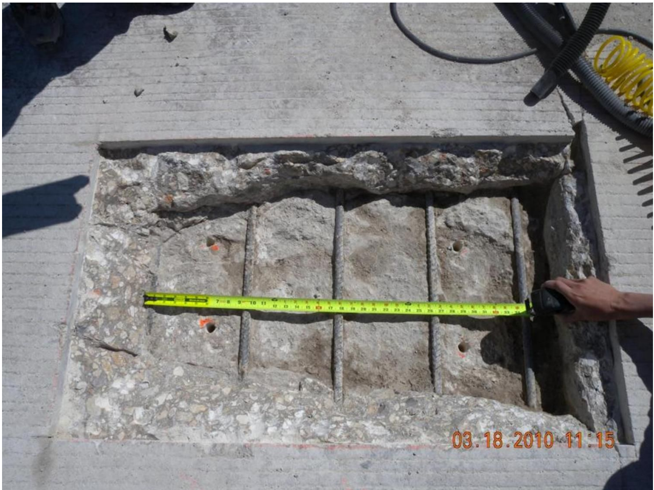
Figure 10-11. Clean repair surfaces.
