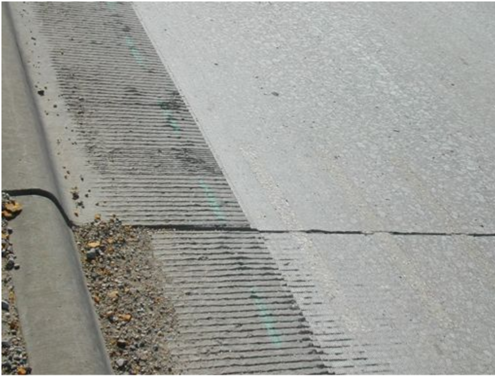
Figure 10-24. After DBR, slab jacking, and diamond grinding of the section shown in Figure 10-17.
