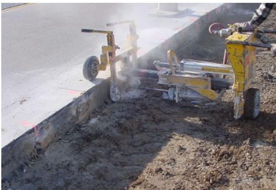
Figure 10-5. Drilling holes at longitudinal joint.
