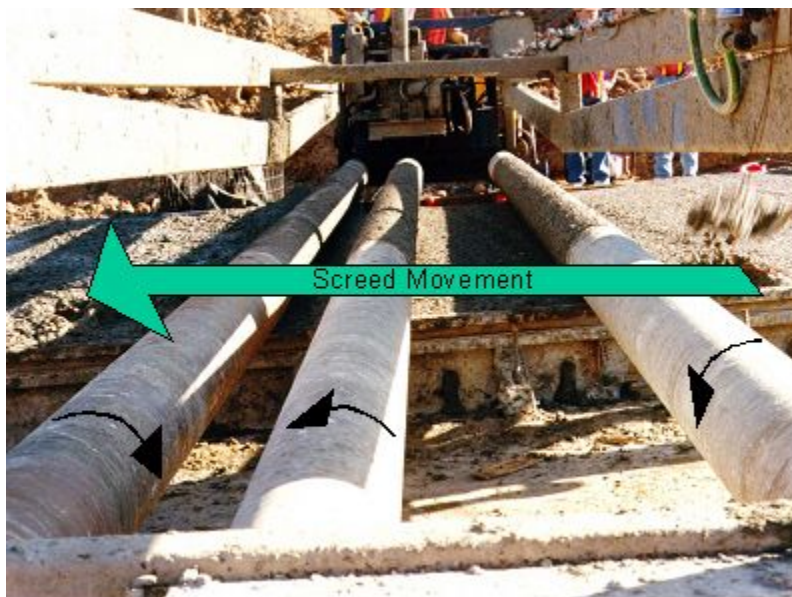
Figure 9-27. A Clary or roller screed.
