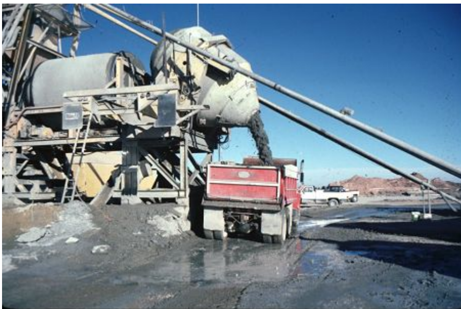
Figure 9-8. Discharging concrete into a dump truck.
