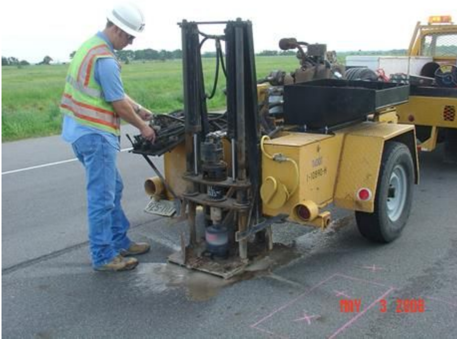
Figure 4-21. Coring using a water-cooled barrel.
