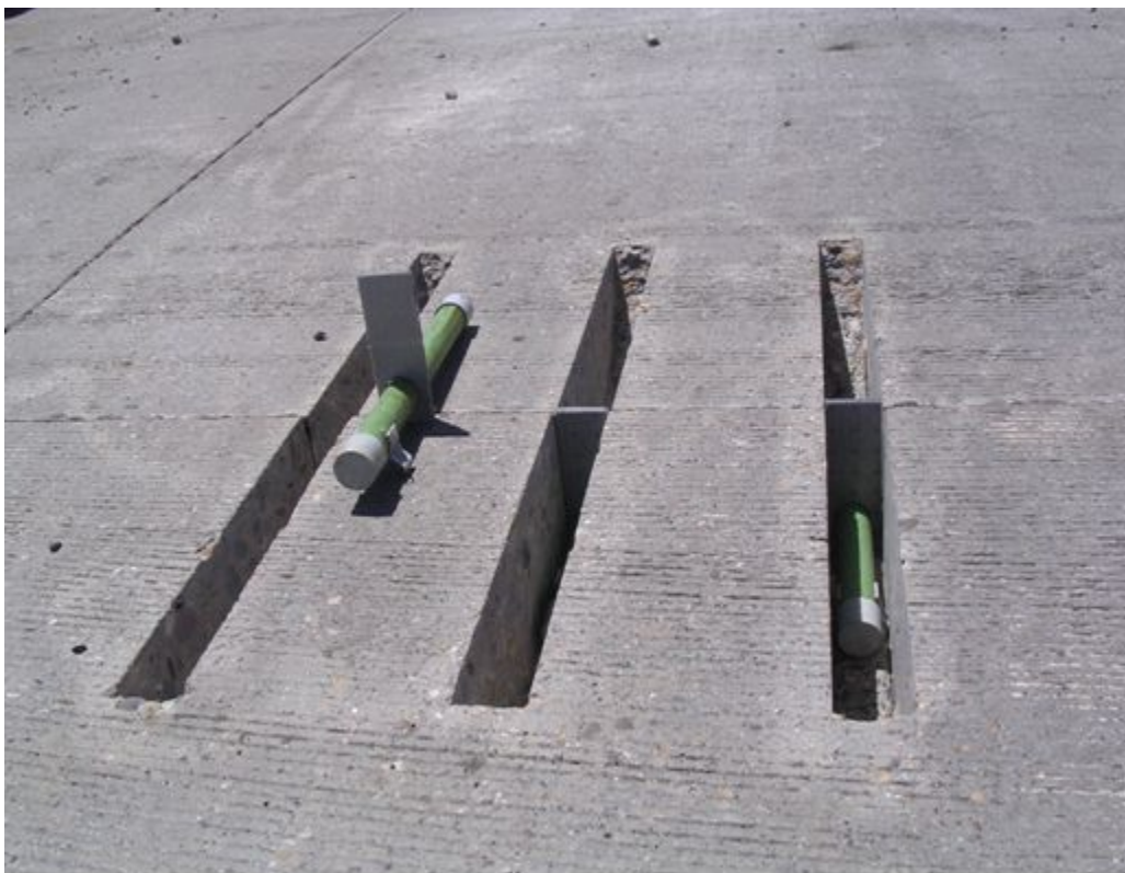
Figure 10-23. Dowel bar in place for backfill material application.
