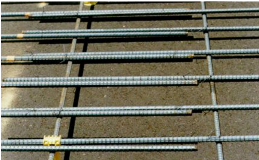
Figure 9-14. Spliced or lapped longitudinal steel.
