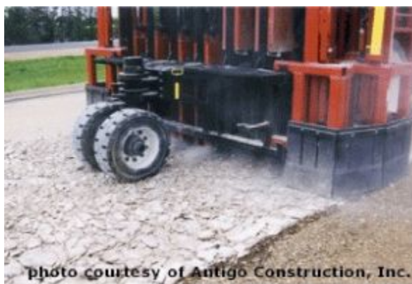
photo courtesy of Antigo Construction, Inc. Figure 7-8. Multi-head Pavement Rubblizer. © Copyright 2006 University of Washington
