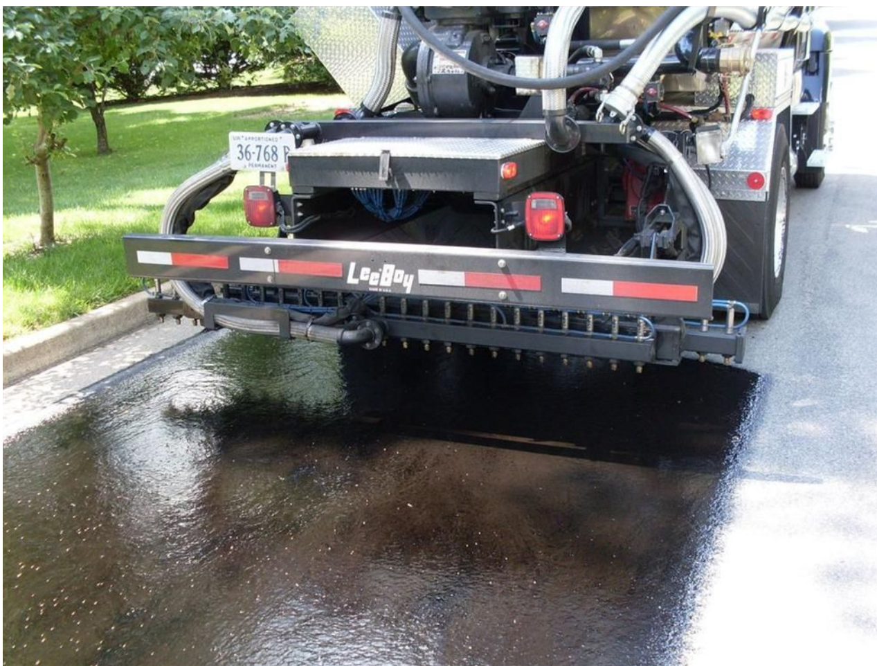
Figure 6-6. Tack Coat Distributor Truck Spray Bar. © Copyright 2006 University of Washington
