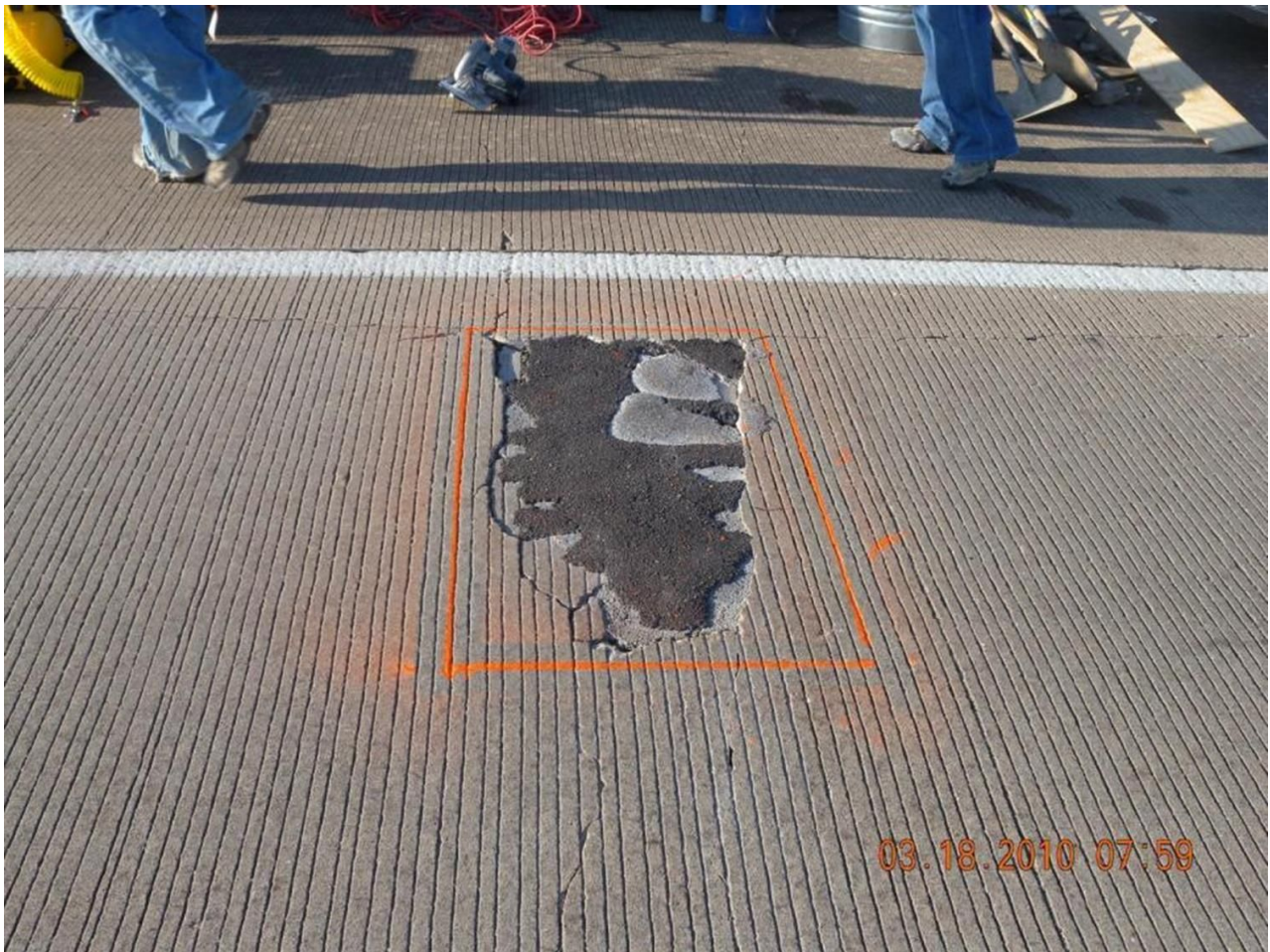
Figure 10-8. Identify the repair limits.
