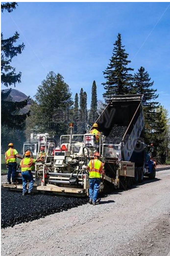
Figure 6-13. End Dump Truck.
