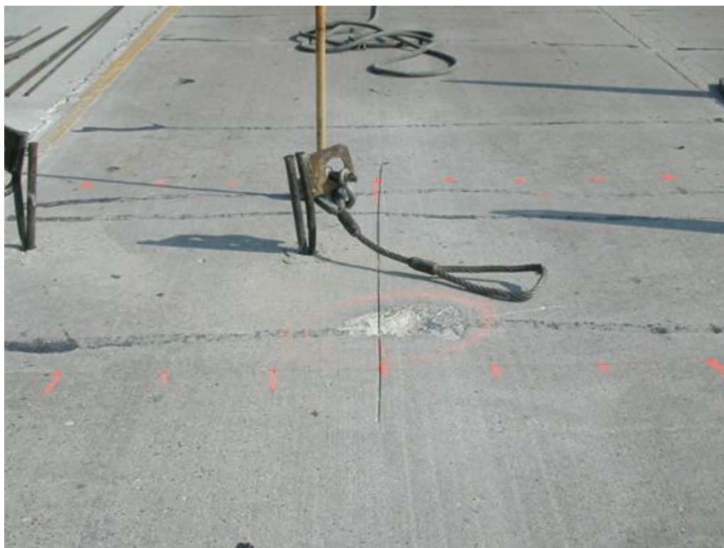
Figure 10-4. Slab ready for lifting.
