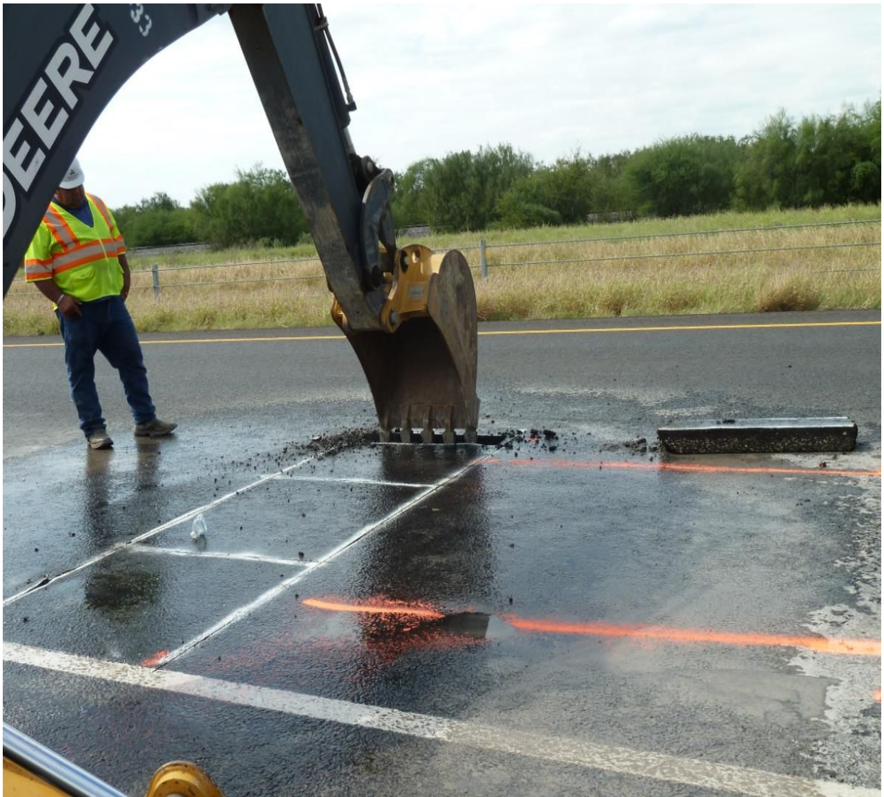
Figure 4-19. Removing hot-mix asphalt (HMA) block with backhoe.
