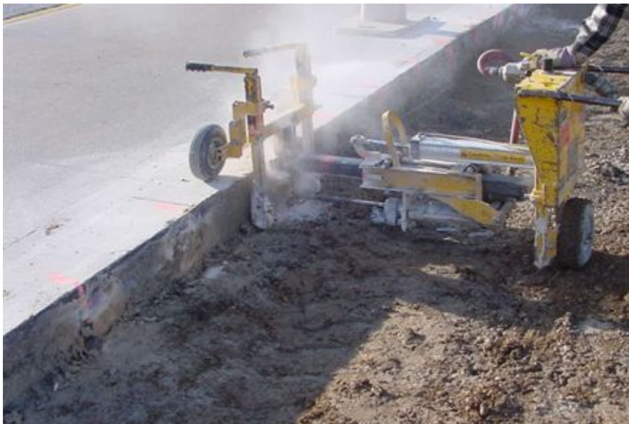
Figure 9-80. Marking and drilling holes at widening joint.
