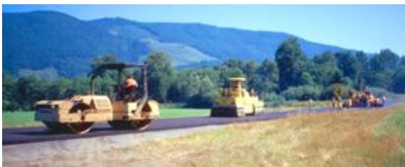
Figure 6-60. Breakdown and Intermediate Rollers. © Copyright 2006 University of Washington
