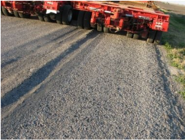
Figure 13-5. Rutting or cracking due to overload of the pavement structure. Recent rainfall or poor drainage conditions resulting in weak or wet subgrade or base materials are often associated with structural damage of this type.
