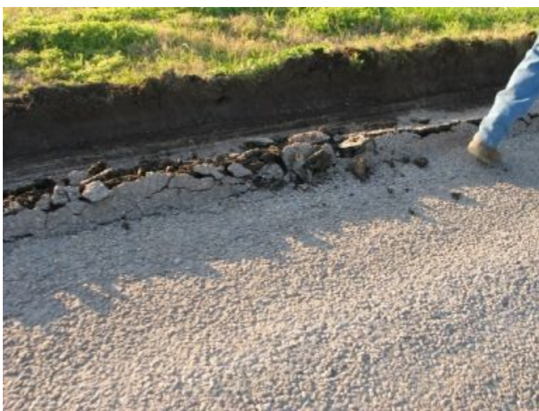
Figure 13-9. Lateral shear failure at the pavement edge (1st photo).
