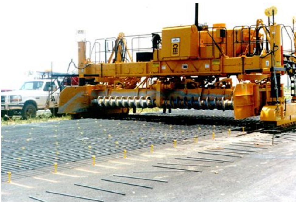
Figure 9-32. Slip-form paver with two augers (idle).
