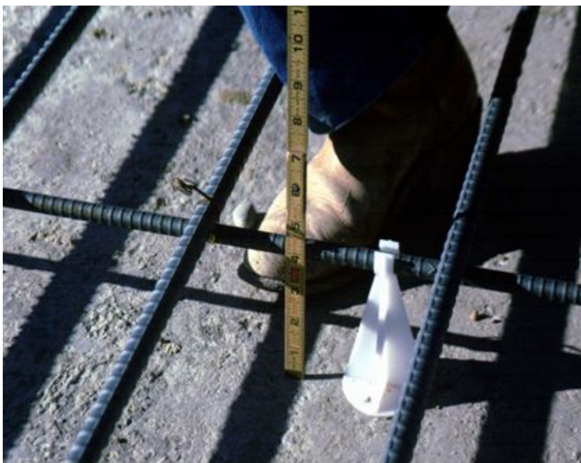
Figure 9-20. Checking steel location.
