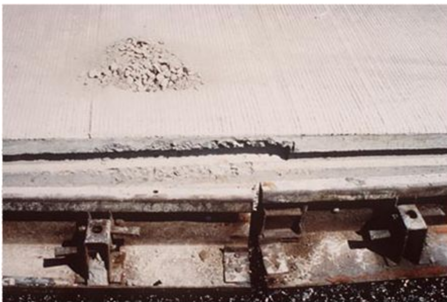
Figure 9-30. Removed side forms.
