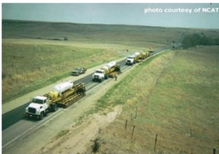
Figure 7-1. Hot In-place Recycling Train.
