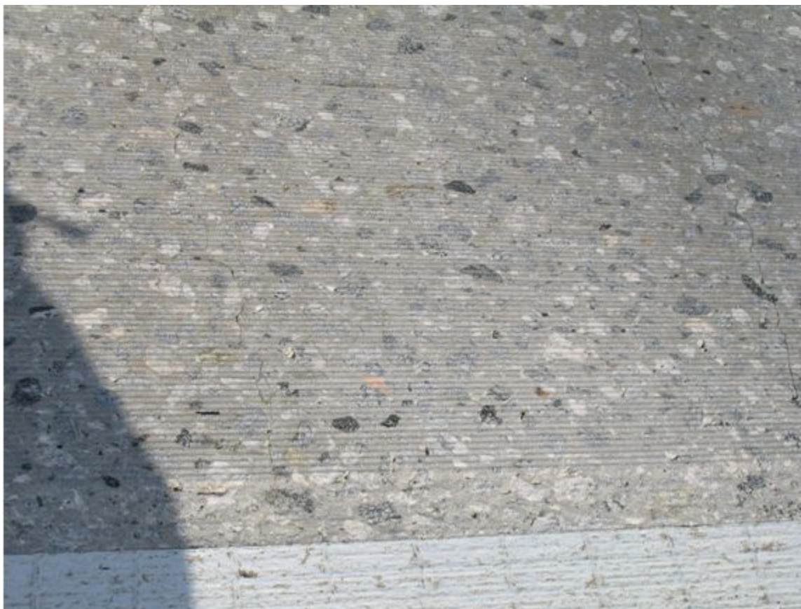
Figure 10-28. Close-up view of diamond ground surface.
