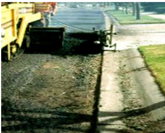
Figure 6-37. Screed Extension. © Copyright 2006 University of Washington
