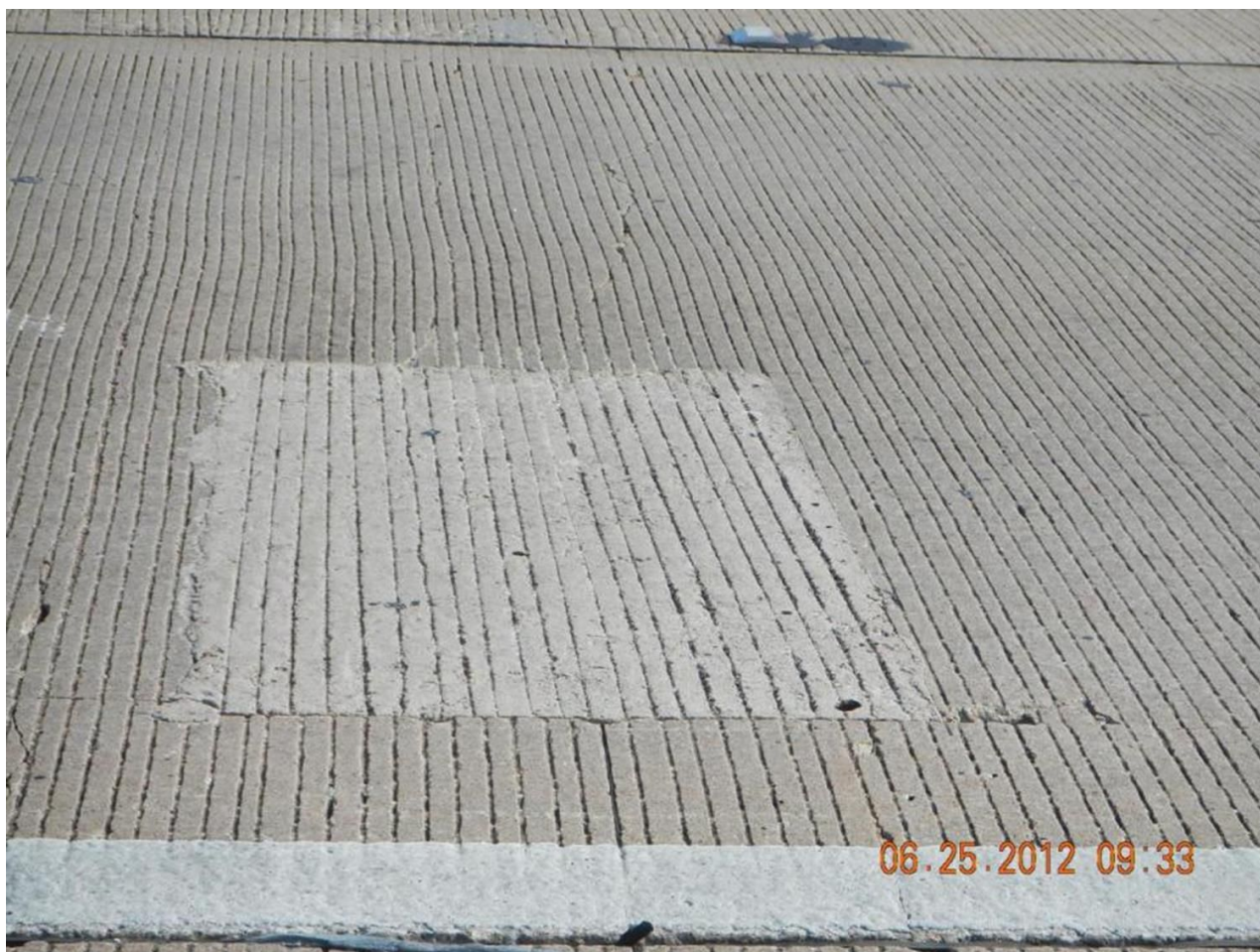
Figure 10-13. Finish the surface.
