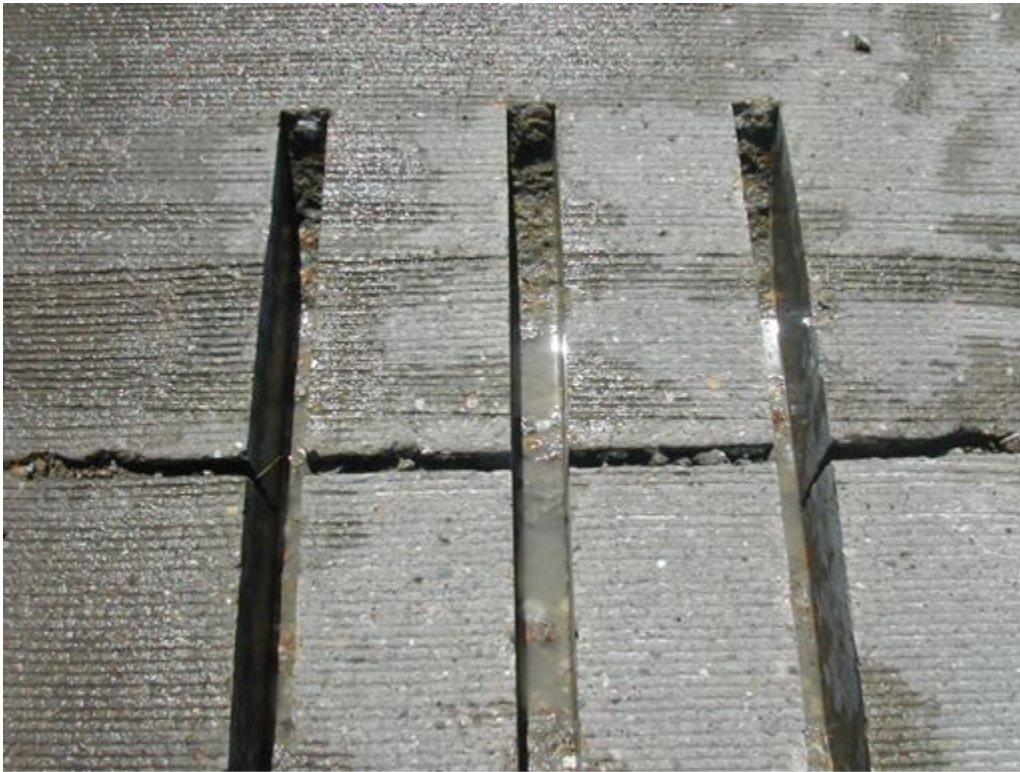
Figure 10-22. Flat bottom after being water cleaned.
