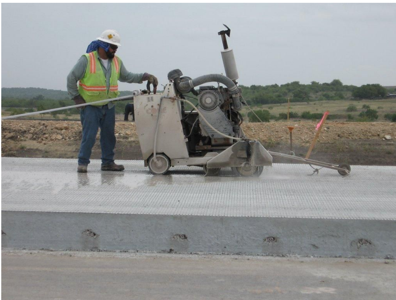
Figure 9-72. Walk-behind saw.
