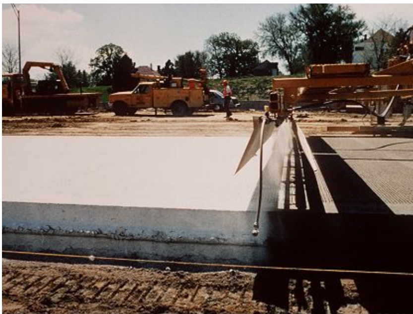
Figure 9-64. Mechanized spraying unit.
