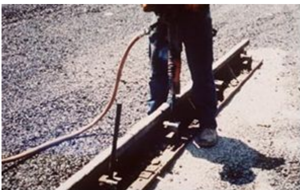
Figure 9-22. Using jackhammer to set staking pin.
