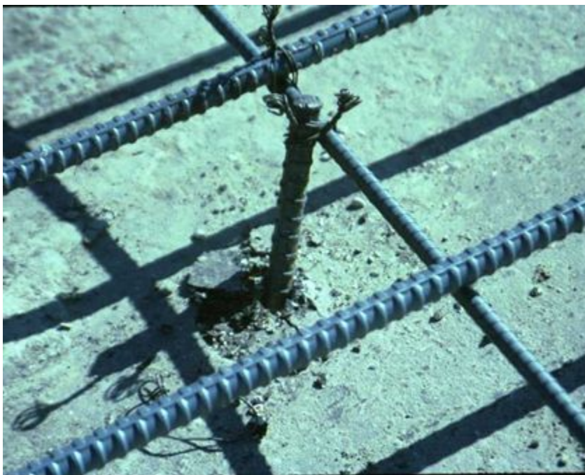
Figure 9-19. Pinning the mat.
