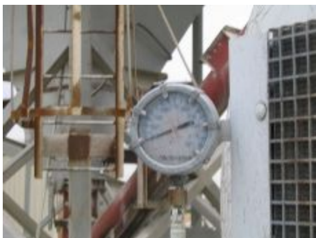
Figure 9-11. Slump meter mounted in the mixing truck.
