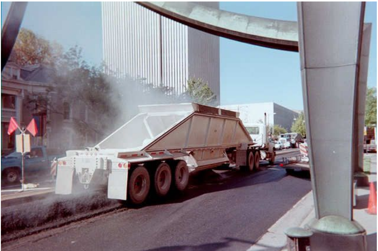
Figure 6-15. Windrow made by emptying a bottom dump truck. © Copyright 2006 University of Washington
