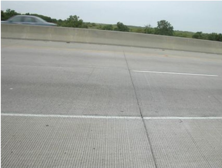
Figure 9-69. Transverse contraction joint.
