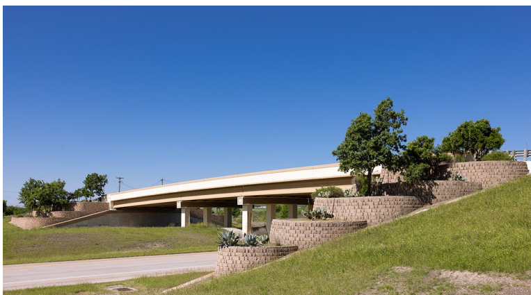
Figure 3-13: Landform modifications at interchanges can reduce the apparent scale of the structure.
