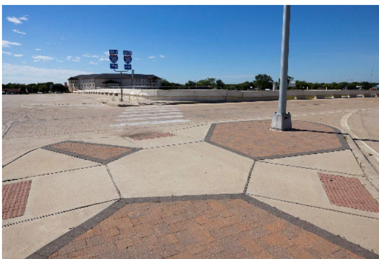
Figure 4-7: Pavers in Traffic Islands
