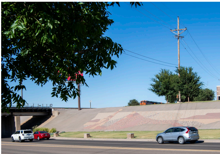
Figure 4-8: Pavers were added to riprap to brighten intersection & add character.
