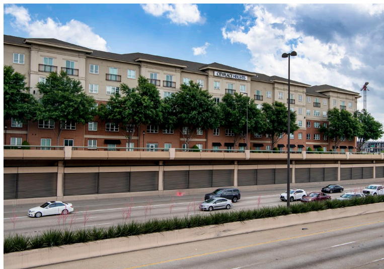
Figure 4-17: Form liners incorporated with architectural details create interesting patterns.
