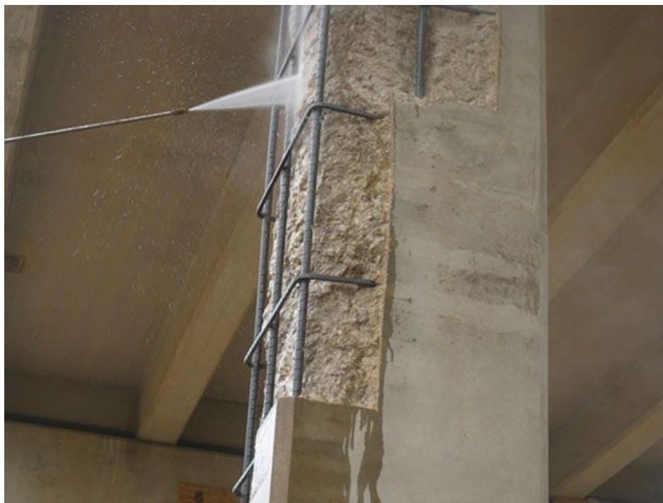
Figure 3-7. Pressurized water to clean and prepare surface (saturated surface dry).
