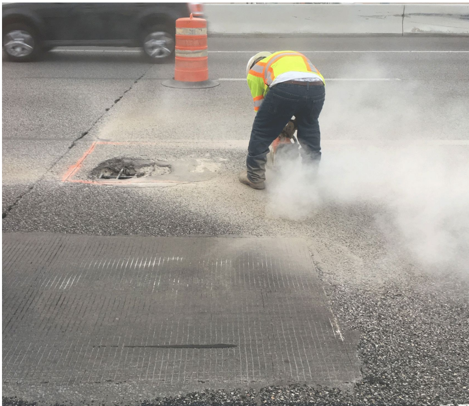
Figure 3-9. Saw-cutting along defined repair boundaries
