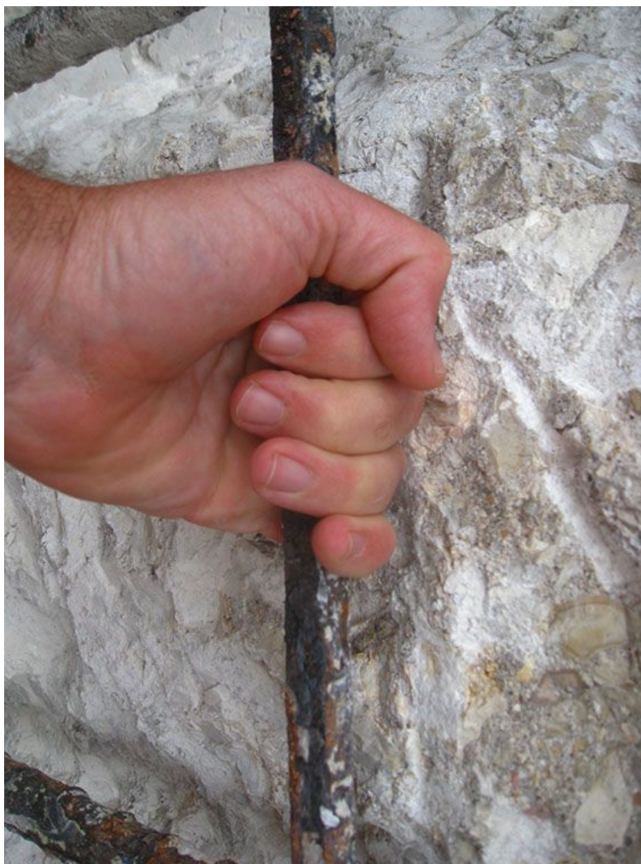
Figure 3-4. Verifying adequate clearance around reinforcing.
