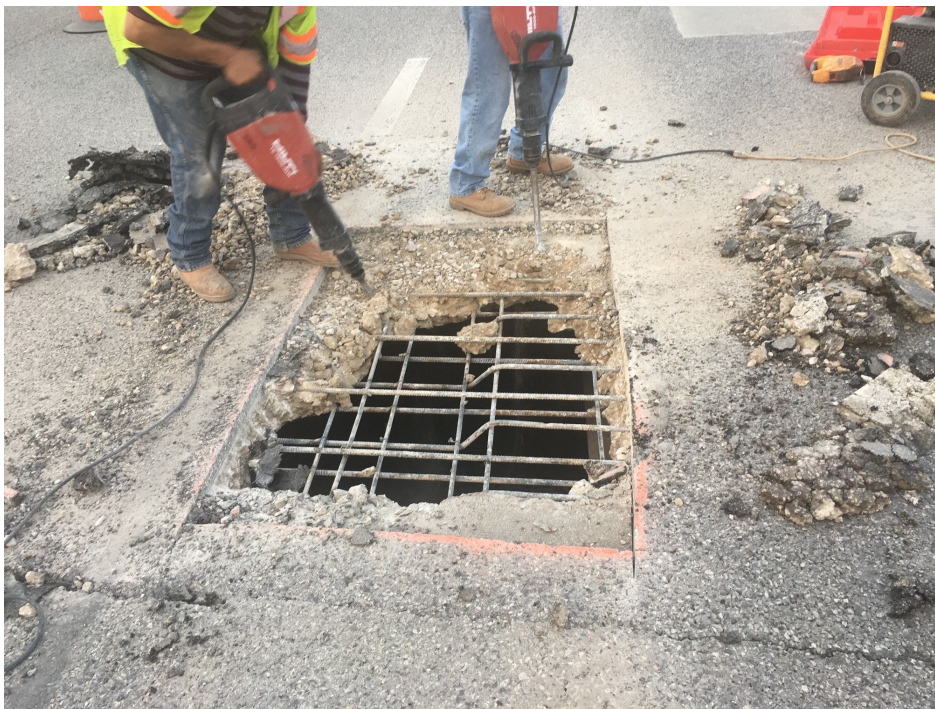
Figure 3-10. Remove deteriorated/unsound concrete
