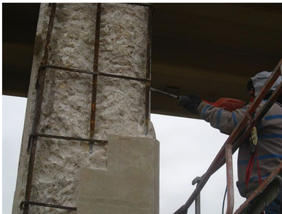
Figure 3-3. Chipping hammer used to remove unsound concrete.
