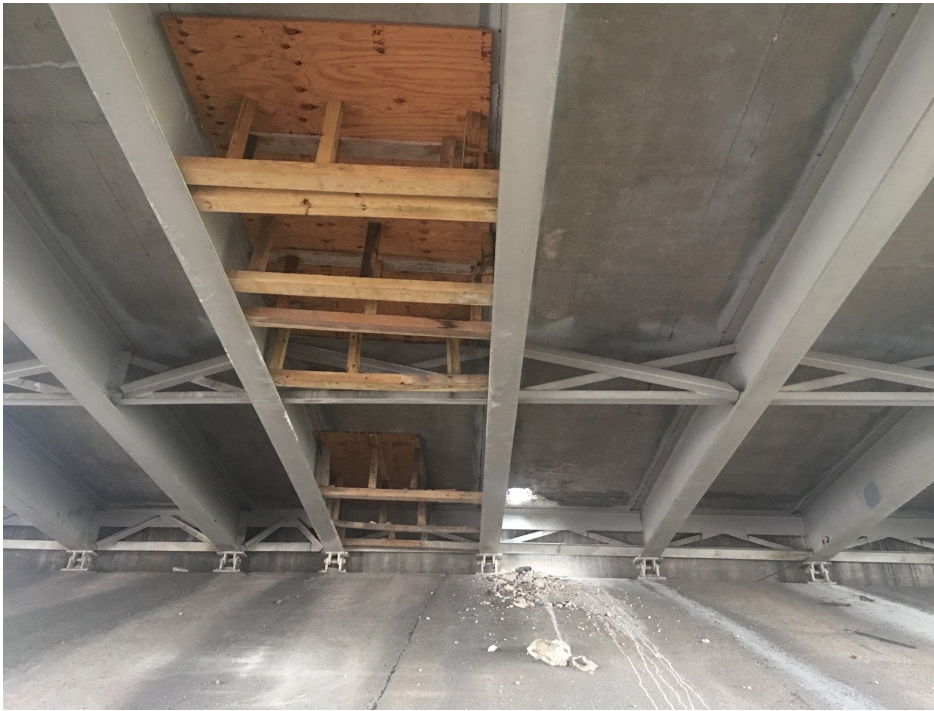
Figure 3-11. Installation of formwork
