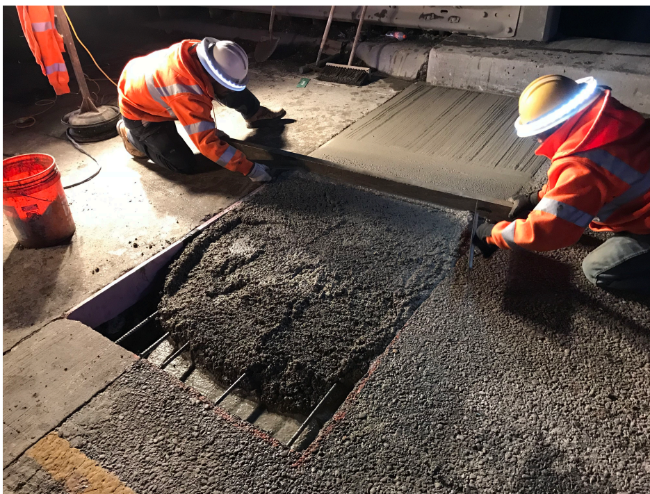
Figure 3-14. Finishing the concrete
