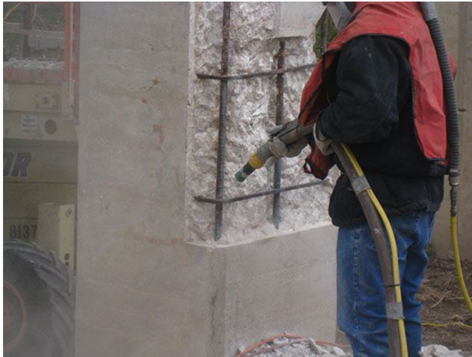
Figure 3-5. Abrasive blasting to clean reinforcing of rust/active corrosion.
