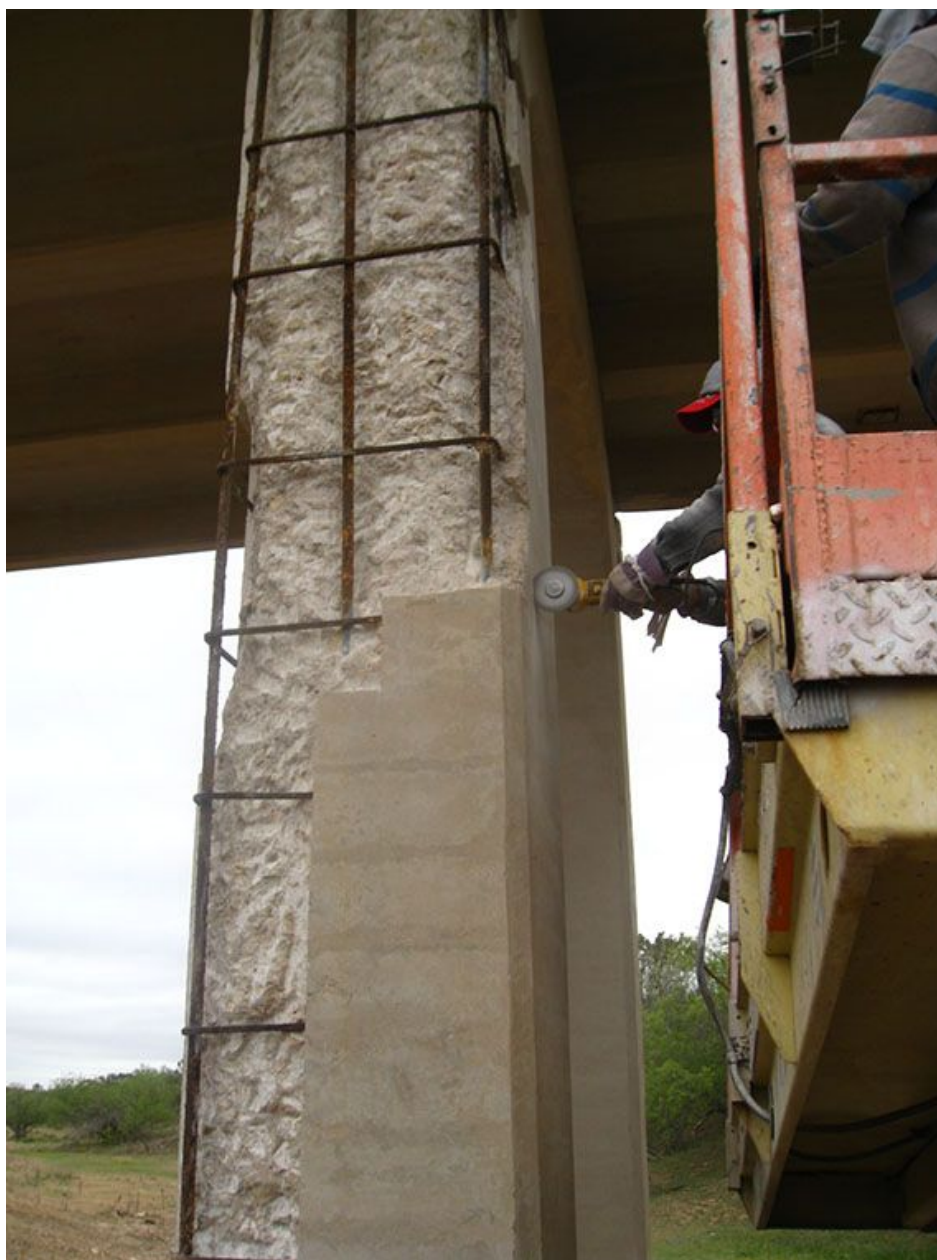
Figure 3-2. Preparation (saw-cutting) straight and squared edges to contain repair material.
