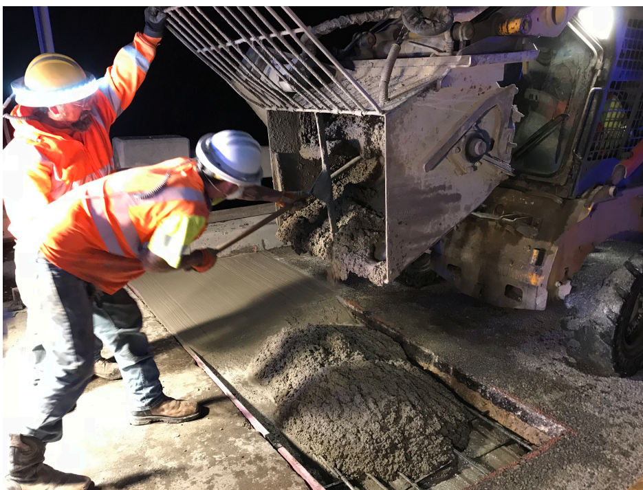
Figure 3-13. Placing the concrete
