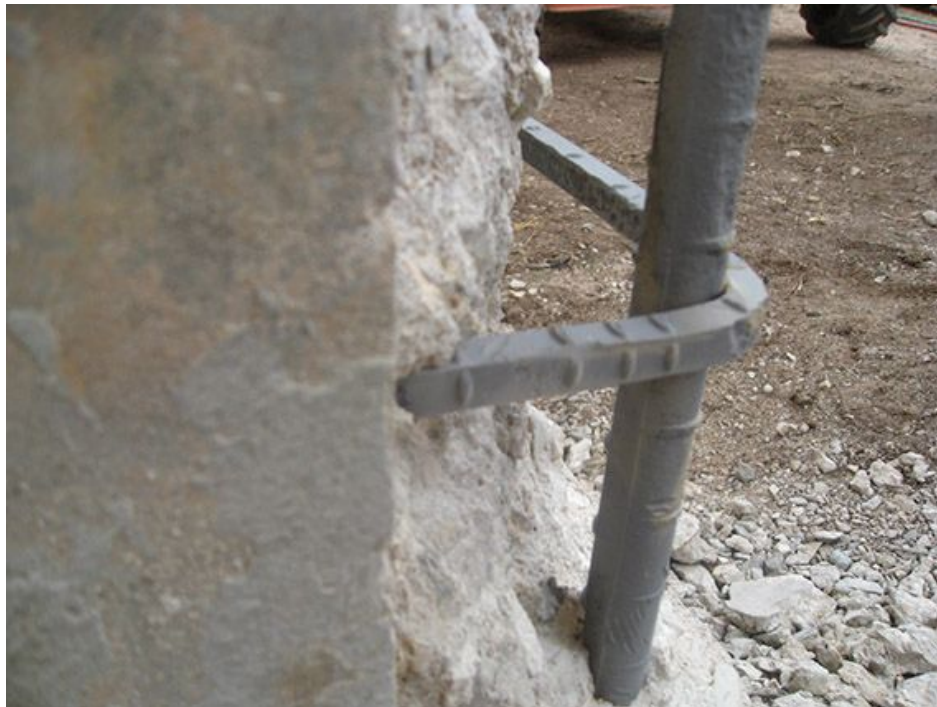
Figure 3-6. Reinforcing cleaned and free of rust.
