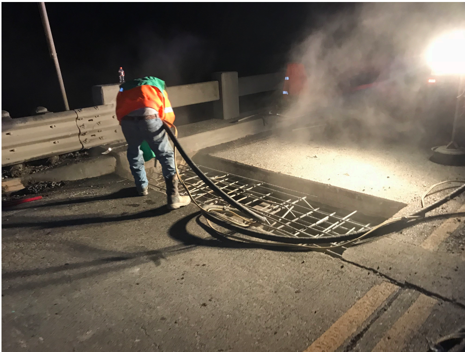
Figure 3-12. Repair area preparation (high-pressure water blasting, or other approved methods to remove dust and debris. Abrasive blasting to remove rust from exposed steel surfaces)
