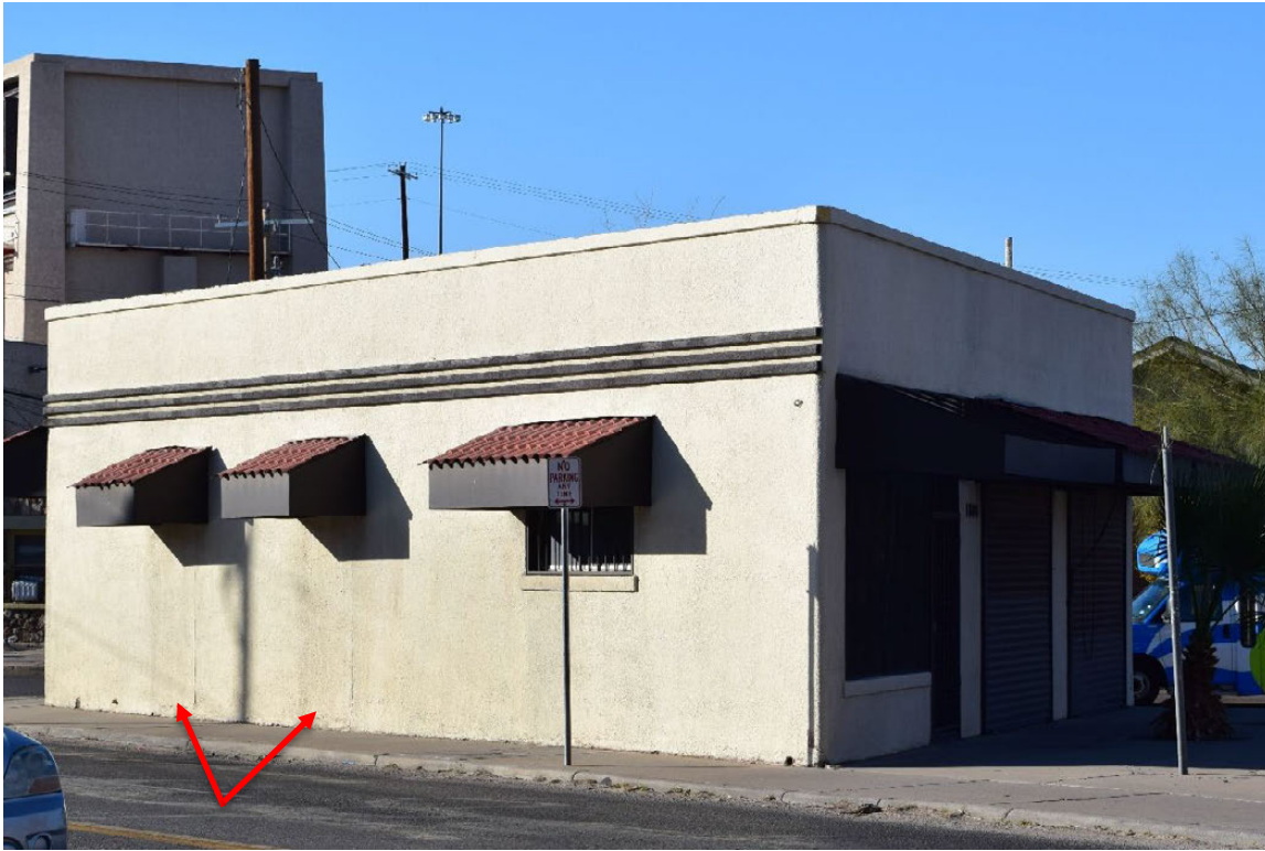
Red arrows note the location of infilled doors, facing west.
