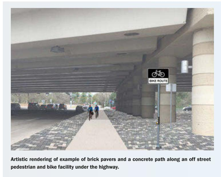
Artistic rendering of example of brick pavers and a concrete path along an off street pedestrian and bike facility under the highway.
