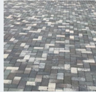
Detail of brick paver layout called herringbone pattern where pavers are laid at 90° angles with an additional brick paver border along the edge, for contrast.
