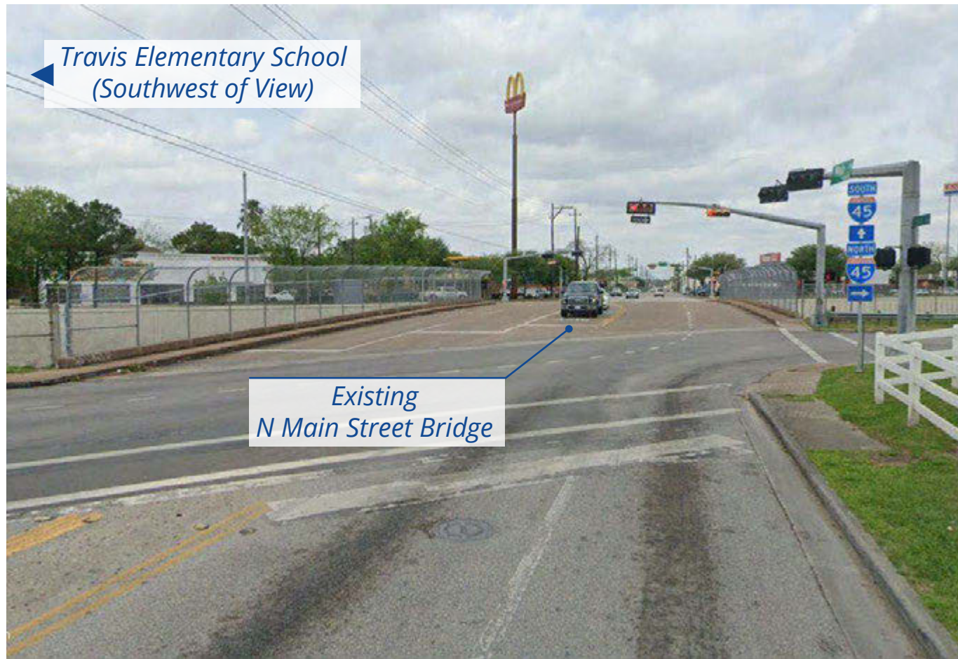
Existing N Main St Bridge over I-45 (Source: Google)
