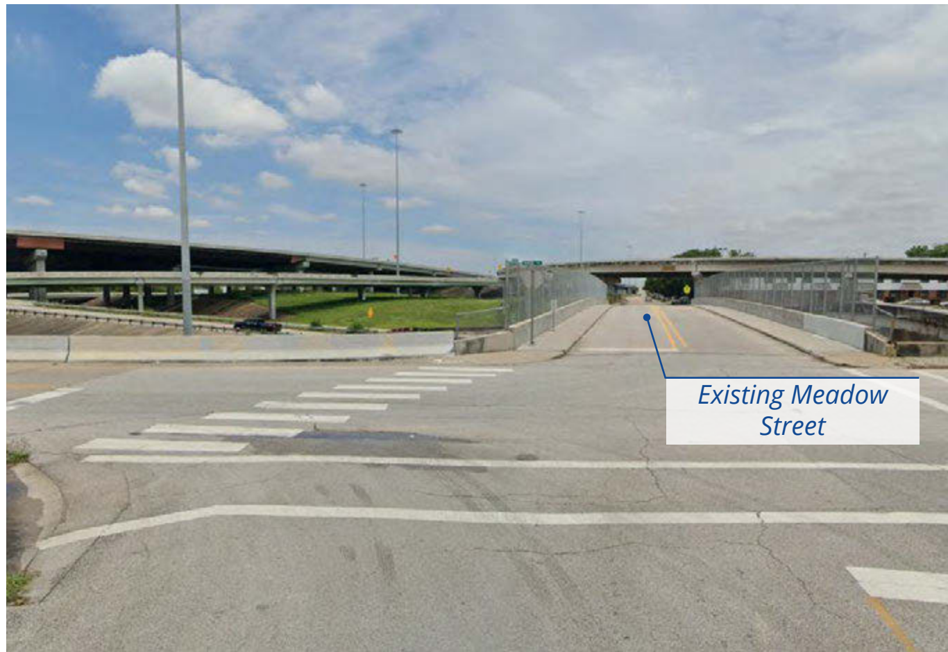
Existing I-10 and Meadow Street
