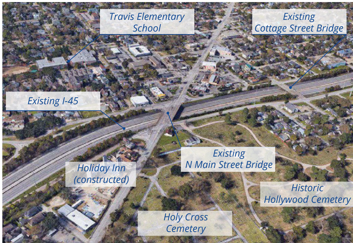
Existing I-45 at Main St and Cottage St (Source: Google)
