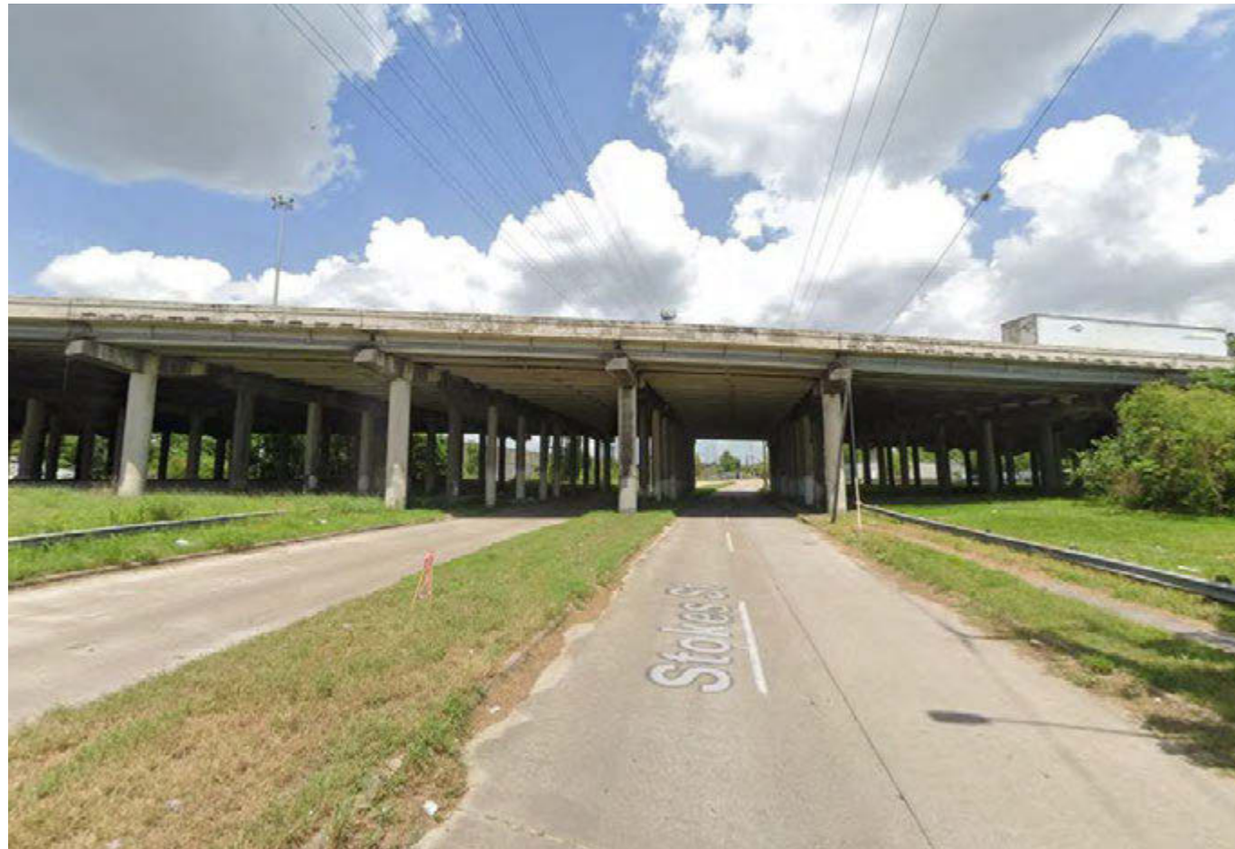
Existing I-45 and Stokes Street
