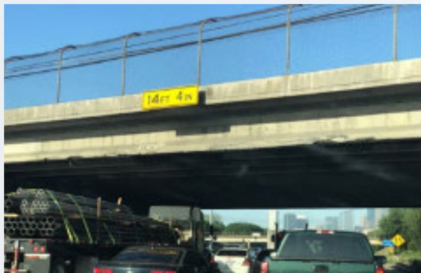
Bridges will be raised to meet national height standards.
