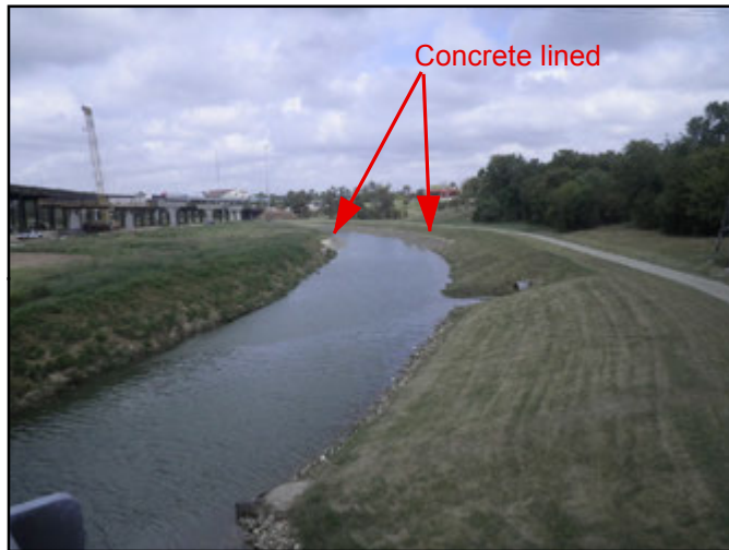
Photo 24 - Looking north from Bicycle Path bridge at White Oak Bayou (concrete lined channel to banks lined with riprap), October 21, 2015
