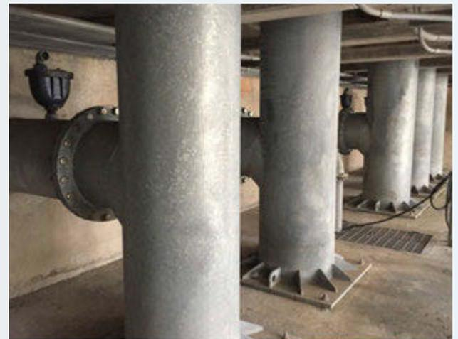
Pump Discharge Pipes.
