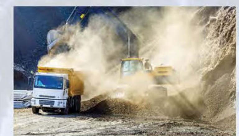
Mitigate Dust & Noise
