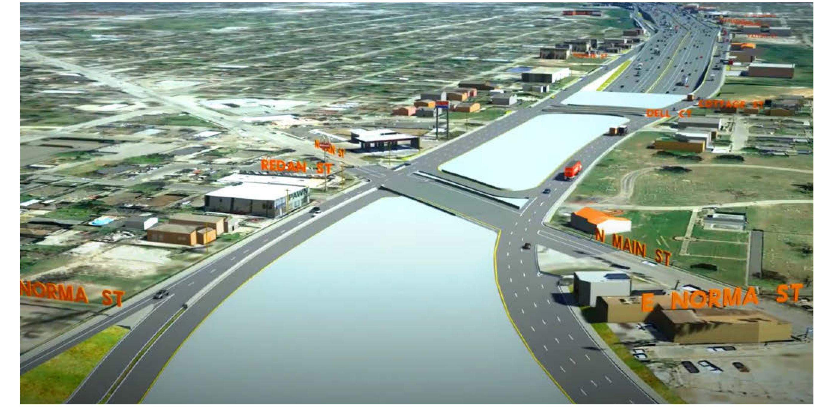
What is a Structural Cap? A structural cap is the concrete infrastructure necessary to build a roadway at natural ground level over a below-grade highway. Beyond its functional purpose, the cap provides an opportunity for the "Art of the Possible." Through public and private funding partnerships, the cap can be transformed into an iconic destination for the community. The exhibits below showcase potential cap features, illustrating how the space can be repurposed to benefit the community.
