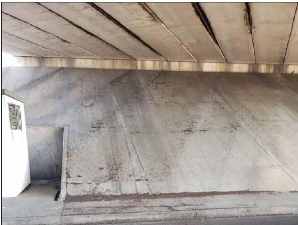
**Photo 14:** View looking south at beneath the bridge at Wells Branch Pkwy. Bat guano along the ground and staining along the expansion joints are visible.
