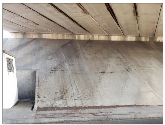
**Photo 14:** View looking south beneath the bridge at Wells Branch Parkway. Bat guano along the ground and staining along the expansion joints are visible. Bats were also observed in the expansion joints.
