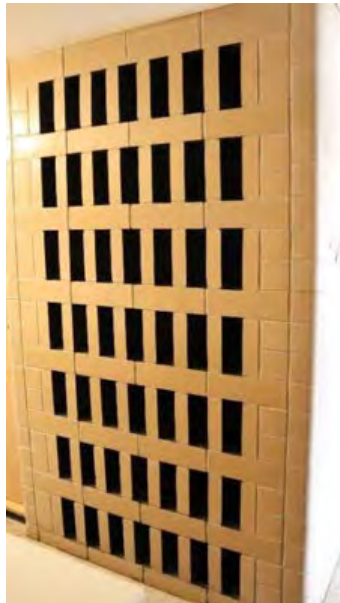
Interior pierced glazed brick wall.
