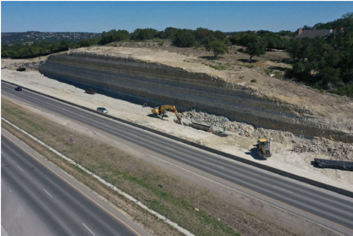
Cliff cuts and utility work along northbound Loop 360
