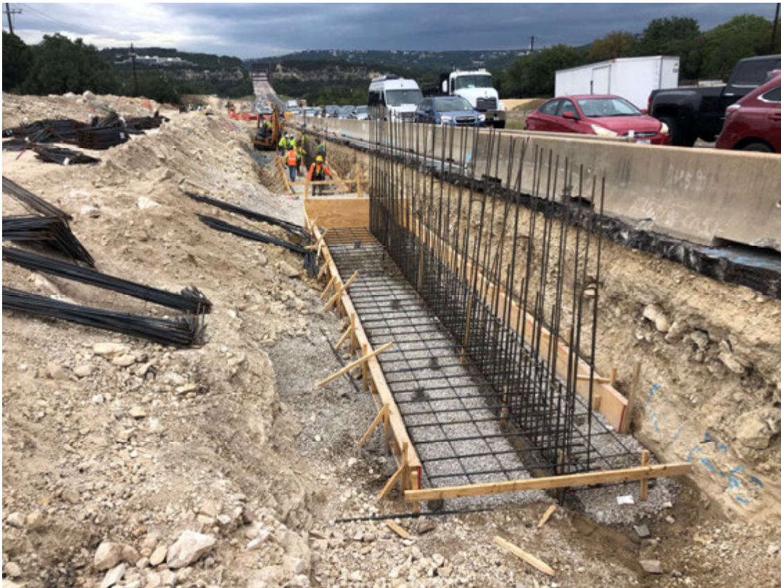
Crews placing a retaining wall along southbound Loop 360 at Riverbend Church
