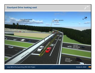
This rendering shows Courtyard Drive looking east. You can see the Loop 360 mainlanes running in either direction underneath the cross street. You will also notice the shared-use path that goes across the north side of the Courtyard Drive bridge, as well as the beginning of the new northbound braided entrance ramp.
