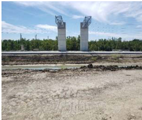
Figure A.6: Ramp 13C in Segment I1A
