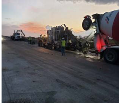
Figure A.7: Kilgore Barrier in Segment I2A1
