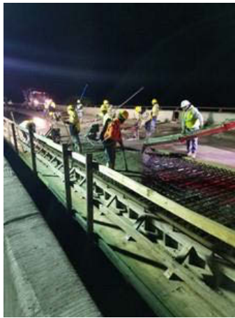
Figure A.8: Bridge 25 Deck Pour in Segment I2B2
