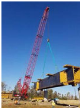
Figure A.5: Bent Cap form at Bridge 10 in Segment I1A
