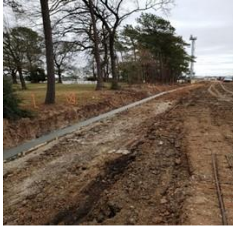
Figure A.7: Retaining Wall Footing in Segment I2B2
