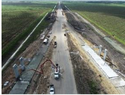
Figure A.4: Toll Plaza Pad being Poured in Segment H2
