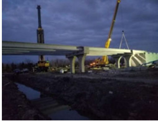
Figure A.7: Beam Installation for Bridge 14 in Segment I2A1
