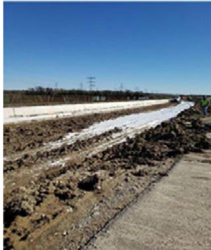
Figure A.8: Lime Placement on Ramp 10 in Segment I2B1
