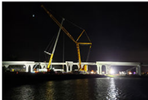
Figure A.4: Beam Installation over US 90 in Segment H2
