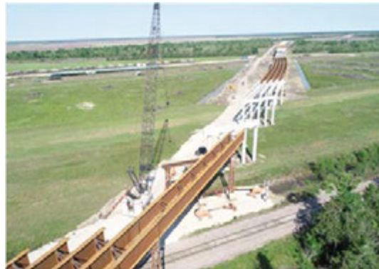
Figure A.5: Bridge 8 Steel Girders in Segment I1A
