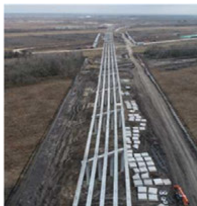
Figure A.6: Bridge 8 Concrete Beams in Segment I1A
