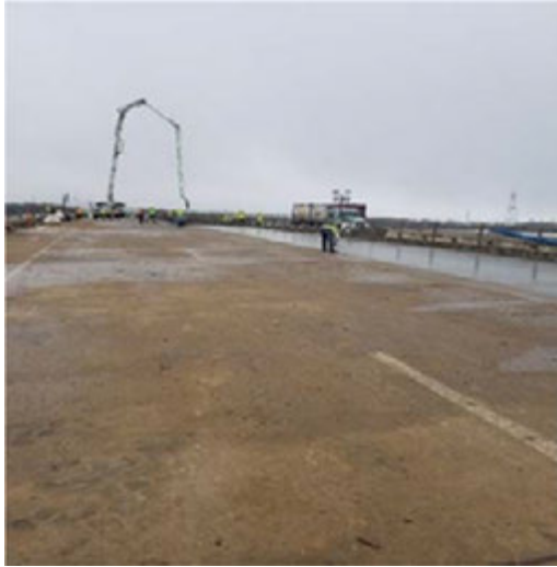
Figure A.10: Deck Pour on Bridge 25 in Segment I2B2
