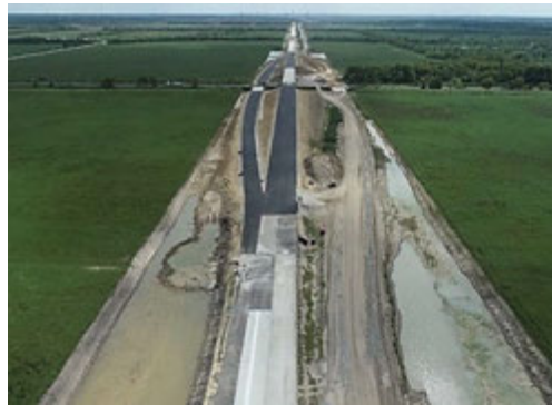
Figure A.5: HMA, Bond Breaker, and CRCP Placement at FM 1414 in Segment I1A
