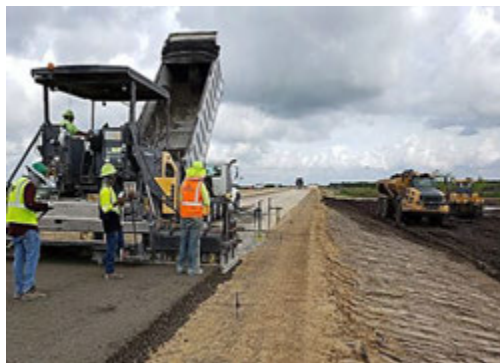
Figure A.5: Embankment and CTB Placement in Segment H2
