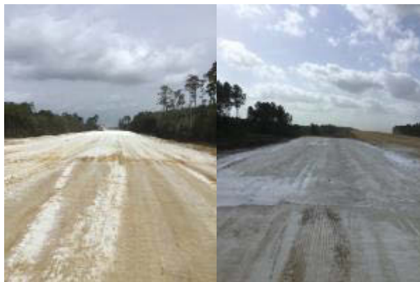
Figure A.3: Lime Remix at a Ramp in Segment H1C
