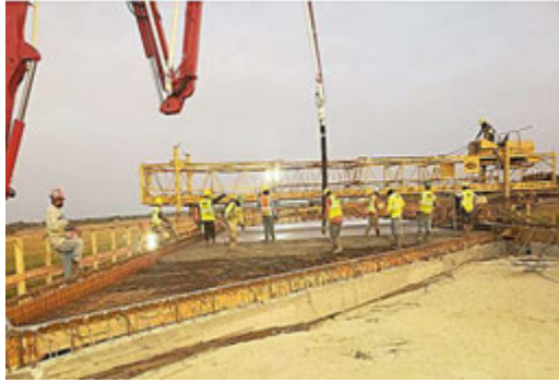
Figure A.4: Bridge 252 Deck Pour in Segment H2
