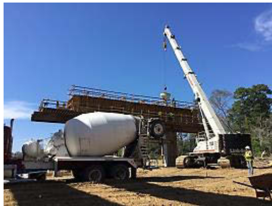
Figure A.2: Bridge 209 Abutment 4 Pour in Segment H1B
