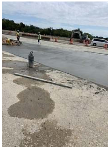
Figure A.11: Concrete Placement at Frontage Road in Segment I2B2
