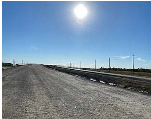
Figure A.8: CTB Placement North of Fisher Road in Segment I2A2
