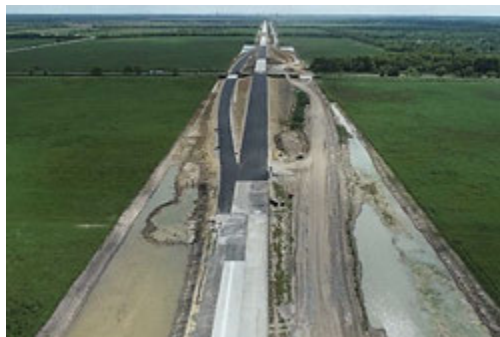
Figure A.6: HMA, Bond Breaker and CRCP Placement at FM 1413 in Segment I1A
