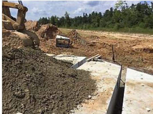
Figure A.1: Backfilling Operations at Culverts in Segment H1A
