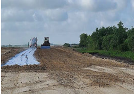
Figure A.10: Liming Operations in Segment I1A
