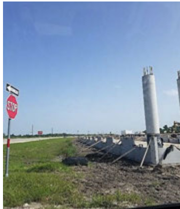
Figure A.11: MSE Panel Installation at Bridge 15 in Segment I2A1
