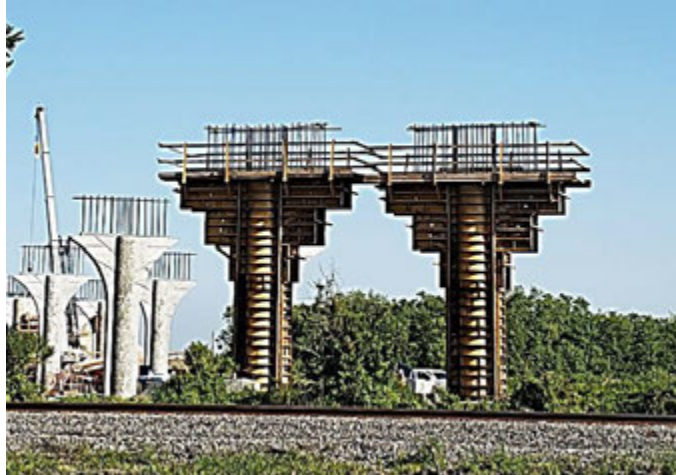
Figure A.7: Column Formwork for Concrete Pour at Bridge 254 in Segment H2
