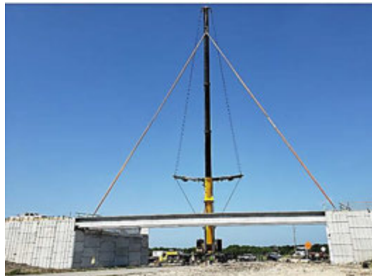
Figure A.9: Beam Erection at Bridge 250 in Segment H2
