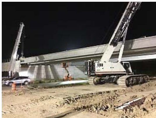
Figure A.5: Girder Launch at Bridge 231 in Segment H1C
