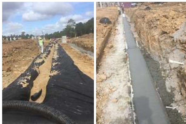
Figure A.2: Leveling Pad for Retaining Wall in Segment H1B
