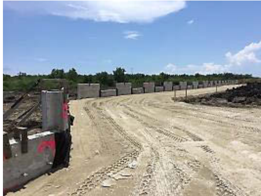
Figure A.4: Backfilling MSE Panels for Retaining Walls in Segment H1C
