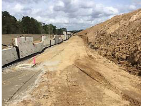
Figure A.1: Setting Deck Panels for Retaining Wall #5 in Segment H1A
