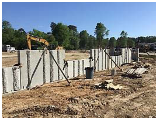
Figure A.6: MSE Panel Installation at Retaining Wall 11 in Segment H1B
