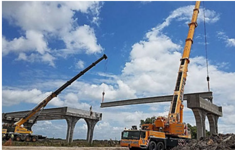
Figure A.8: Beam Installation at Bridge 7A in Segment I1A
