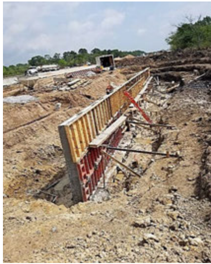
Figure A.14: Culvert Headwall Installation in Segment I2B2
