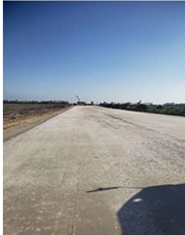
Figure A.7: CTB Placement in Segment I1A
