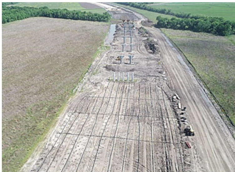
Figure A.9: Wick Drain Placement in Segment I1A
