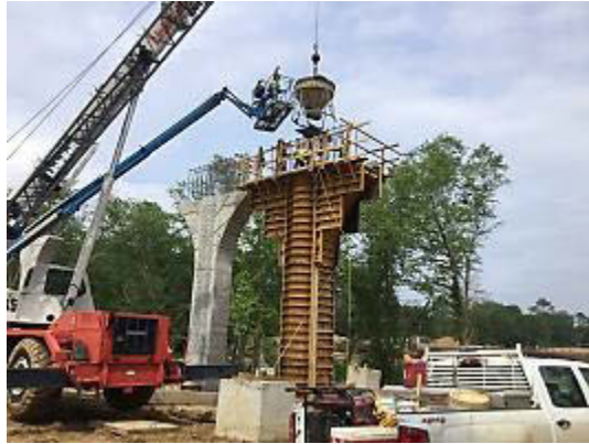
Figure A.4: Concrete Placement for Bent 8 at Bridge 219 in Segment H1B
