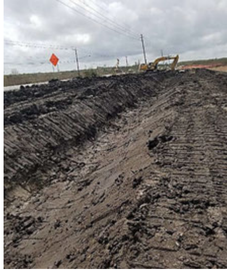
Figure A.10: Grading for Temporary Drainage in Segment I1B
