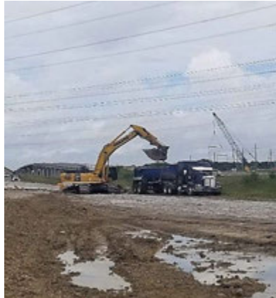
Figure A.11: Existing Eastbound Mainlane Pavement Demolition in Segment I2B1
