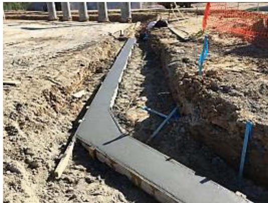
Figure A.5: Level Pad at Retaining Wall 9 in Segment H1B
