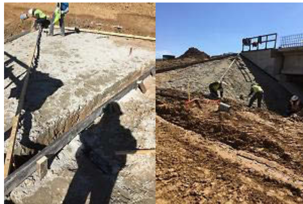
Figure A.2: Forming for Rip Rap placement at Bridge 202 in Segment H1A
