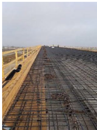
Figure A.12: Deck Rebar installation at Bridge 15 in Segment I2A1
