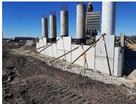
Figure A.8: MSE Construction at Bridge 250 in Segment H2
