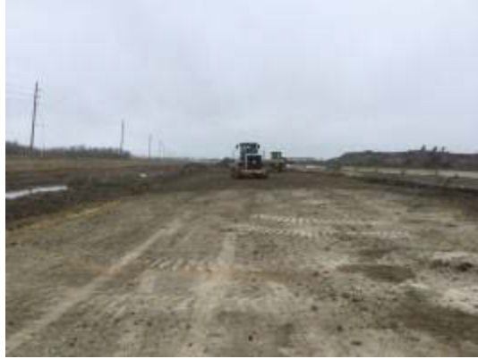
Figure A.13: Lime Stabilized Embankment Construction at Ramp 16 in Segment I2A1
