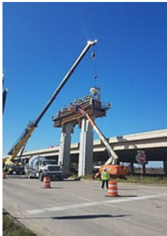
Figure A.11: Bent Cap Construction at Bridge 15 in Segment I2A1
