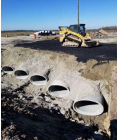
Figure A.7: RCP Installation at FM686 Crossing in Segment H2
