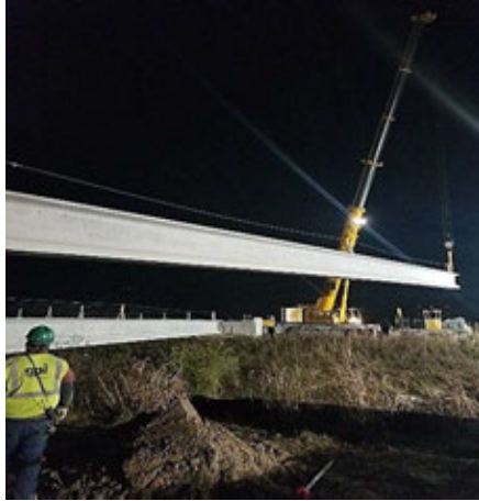
Figure A.10: Beam Placement at Bridge 4A in Segment I1A
