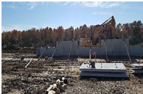
Figure A.15: MSE Panel Placement for Retaining Wall 22 in Segment I2B2
