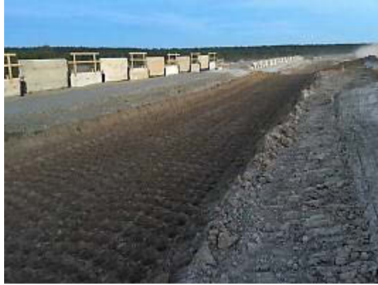
Figure A.4: Placement of MSE Panels at Retaining Walls 17, 18 & 19 in Segment H1C
