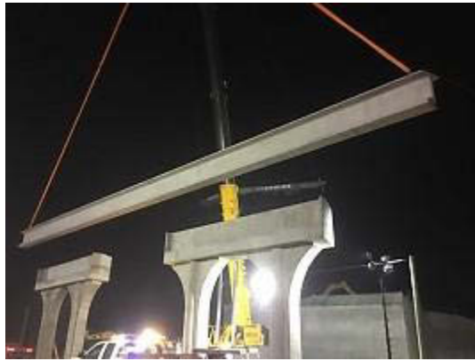
Figure A.1: Nighttime Beam Placement at Bridge 206 in Segment H1A
