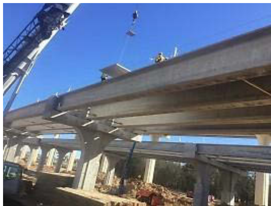
Figure A.3: Setting Deck Panels for Span 3 at Bridge 203 in Segment H1A
