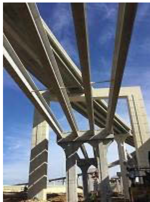
Figure A.2: Beam Placement at Bridge 204 in Segment H1A
