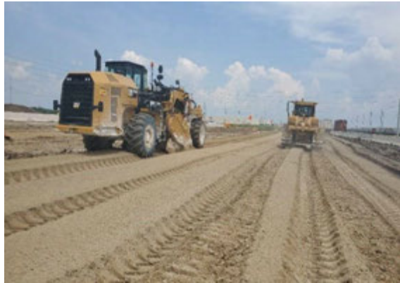
Figure A.8: Embankment Construction East of FM 1405 in Segment I-2B1
