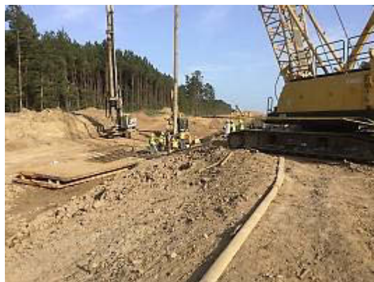
Figure A.3: Drilled Shaft Construction at Bridge 236, Bent 5 in Segment H-1C
