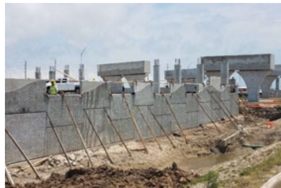
Figure A.9: MSE Wall Construction at FM1405 in Segment I-2B1
