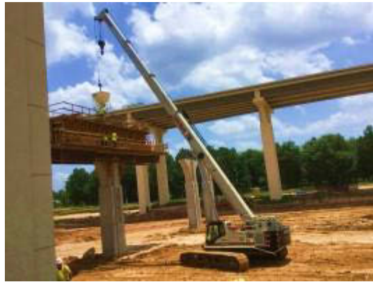
Figure A.1: Concreting Operations at Bridge 203 in Segment H-1A
