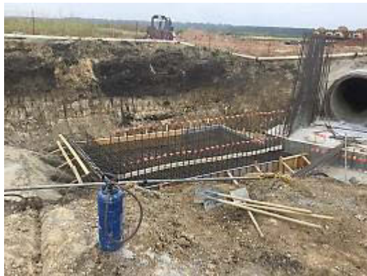
Figure A.5: Wing Wall at Luce Bayou in Segment H-1C
