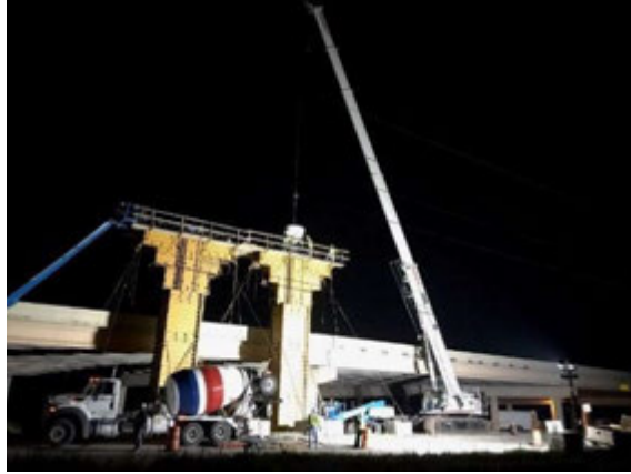
Figure A.7: Column Construction at Bridge 15, Bent 15 in Segment I-2A1
