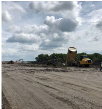
Figure A.6: Embankment Construction in Segment I-1A
