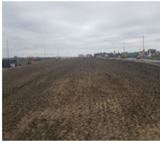
Figure A.8: Embankment Construction West of FM 1405 in Segment I-2B1
