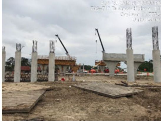
Figure A.10: View of Bridge Construction at SH 146 in Segment I-2B2
