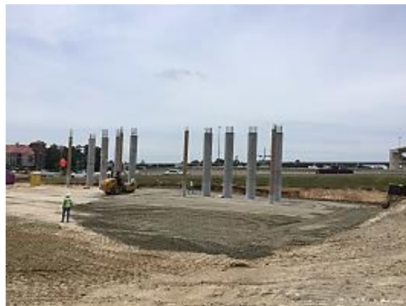
Figure A.3: Bridge 203 and 204 Embankment in Segment H-1A
