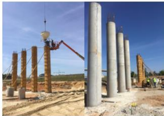
Figure A.2: Bridge 203, Concrete Pour at Abutment Extensions in Segment H-1A
