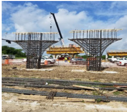
Figure A.9: Bridge 22, View of Bent Construction in Segment I-2B2
