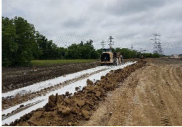
Figure A.7: Embankment Lime Operations in Segment I-2B1
