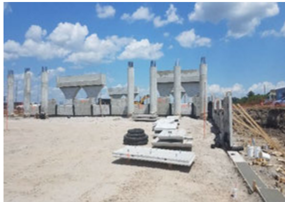
Figure A.6: MSE Wall Construction at FM 1405 in Construction Segment I-2B1
