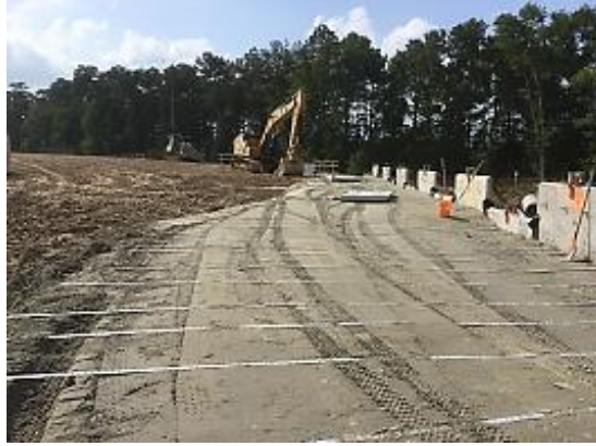
Figure A.4: View of MSE Wall #08 Installation in Segment H-1A
