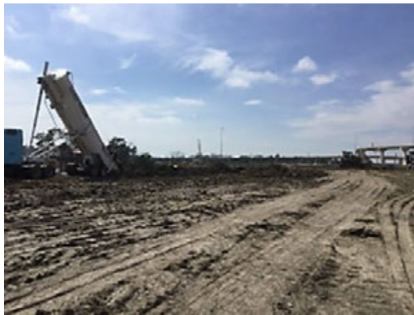
Figure A.1: Embankment Between US-59 201 and Loop 494 in Segment 1
