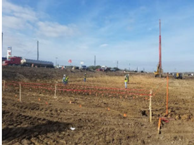
Figure A.13: Bridge 20, Wick Drain Installation in Segment 3
