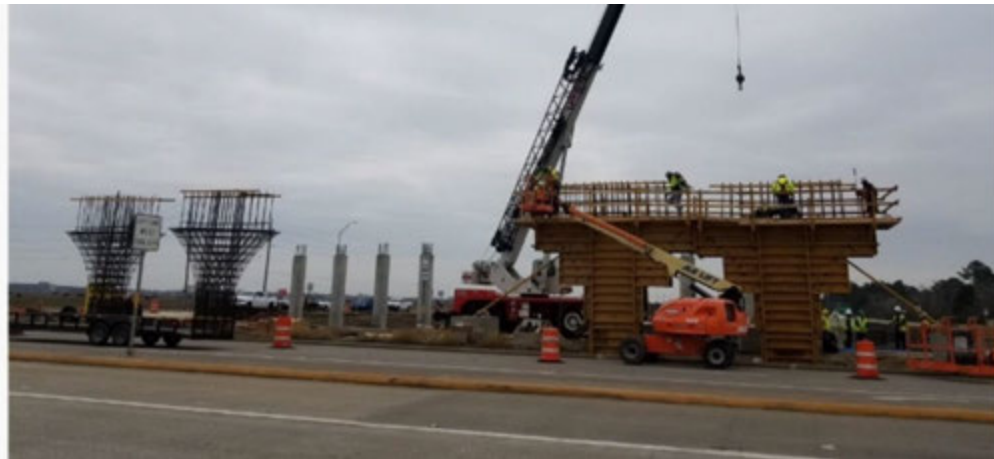
Figure A.14: Bridge 20, Column Construction in Segment 3
