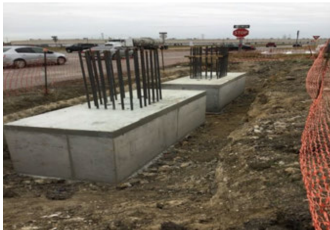
Figure A.12: Bridge 20, View of Constructed Footings in Segment 3
