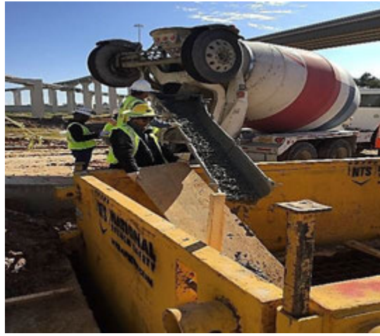
Figure A.4: Bridge 203, Bent 3, Concrete Pour for the Footing in Segment 1
