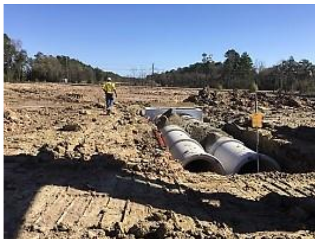
Figure A.9: Drainage Between US-59 and Loop 494 in Segment 1
