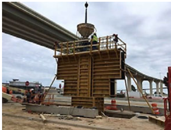
Figure A.5: Bridge 203, Bent 2, Concrete Pour at Column 1 in Segment 1
