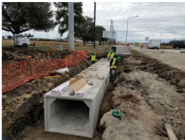
Figure A.15: Culvert installation at Eastbound Frontage Road Segment 3
