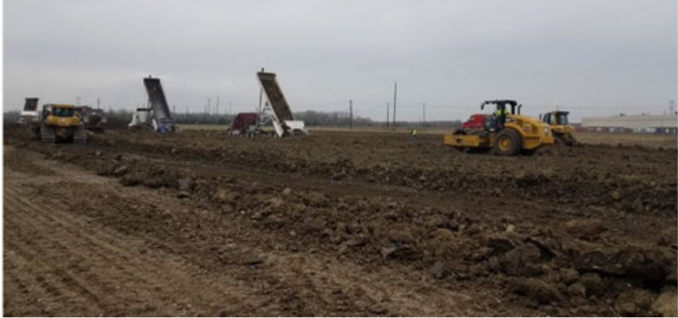
Figure A.10: View of Earthwork Operations in Segment 1
