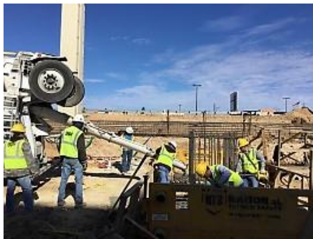
Figure A.6: Bridge 203, Bent 6, Concrete Pour at Footing in Segment 1
