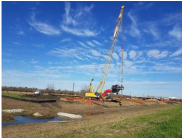
Figure A.11: Bridge 15, Drilled Shaft Construction in Segment 3
