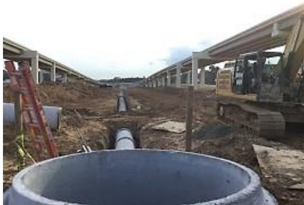
Figure A.8: View of Drainage Installation West of US-59 in Segment 1
