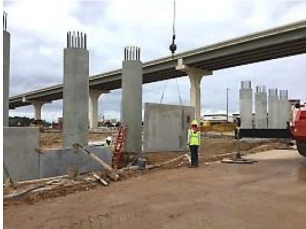
Figure A.7: View of MSE Wall Installation in Segment 1
