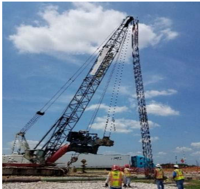
Figure A.11: Bridge 20, Abutment 1 Installation of Drilled Shaft Cage in Segment 3
