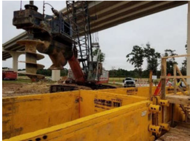
Figure A.8: Bridge 204, Drilled Shaft Construction in Segment 1
