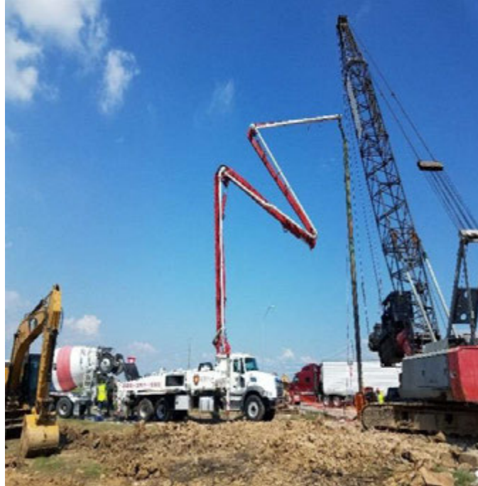
Figure A.12: Bridge 20, Abutment 4 Drilled Shaft Construction in Segment 3
