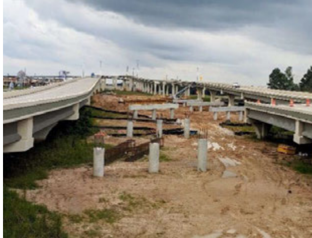
Figure A.7: Bridges 201 and 202, View of Columns and Bent Caps in Segment 1
