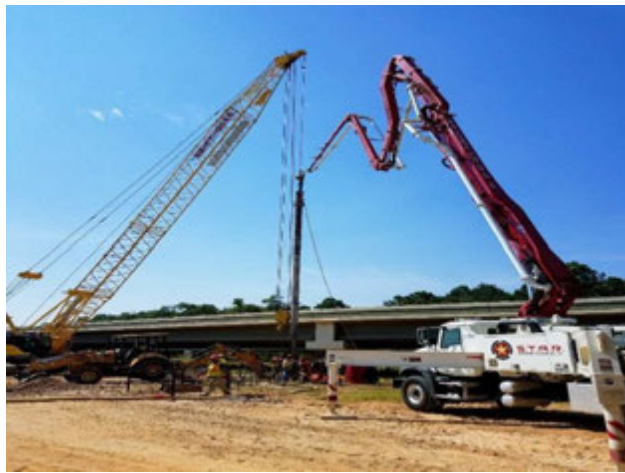
Figure A.6: Bridge 202, Bent 5 Concrete Pour at Drilled Shaft in Segment 1
