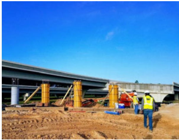
Figure A.2: Bridge 201, Bent 3 Drilled Shafts in Segment 1
