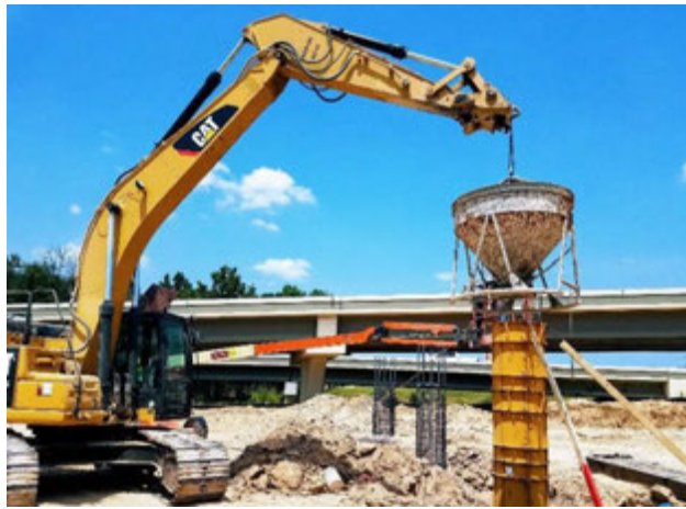
Figure A.3: Bridge 201, Bent 3 Concrete Pour for Columns in Segment 1
