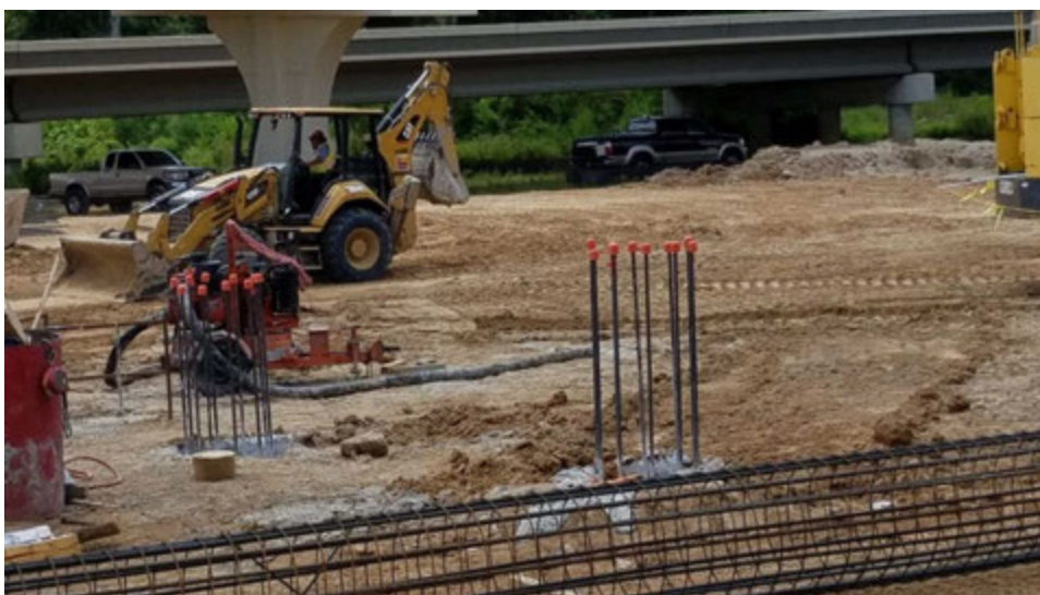
Figure A.2: Drilled Shaft Construction at Bridge 201 in Segment H
