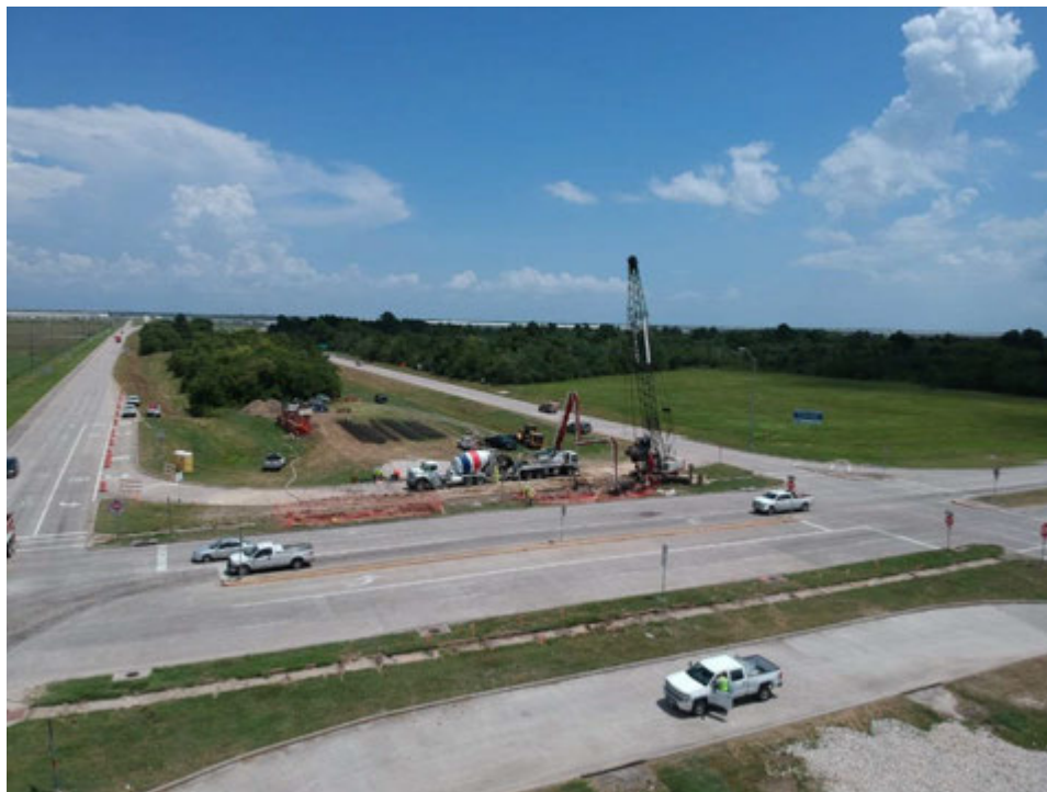
Figure A.8: Drilled Shaft Construction at Bridge 20 (FM 1405) in Segment I-2B
