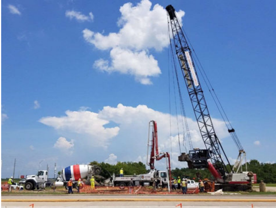
Figure A.7: Drilled Shaft Construction at Bridge 20 (FM 1405) in Segment I-2B
