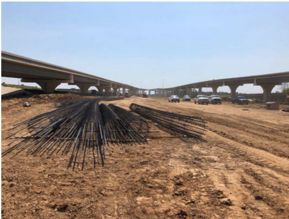
Figure A.6: Drilled Shaft Rebar at Bridges 201 and 202 in Segment H
