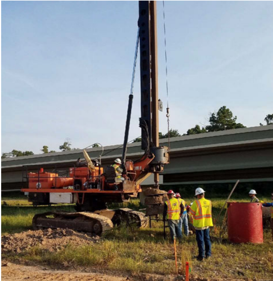
Figure A.1: Drilled Shaft Construction at Bridge 201 in Segment H
