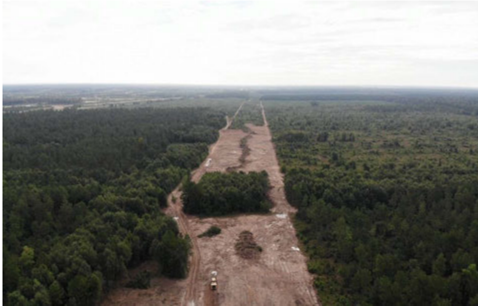
Figure A.3: View of Clearing and Grubbing in Segment H looking East
