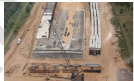
Segment E Morton Road Interchange
