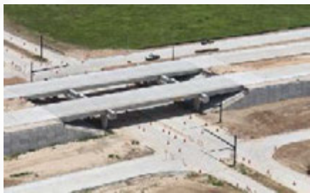
Segment E Bridgeland Creek Parkway Interchange
