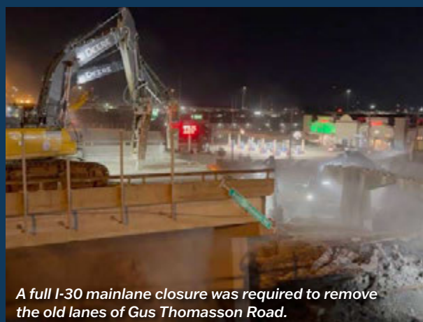
Full removal of the old Gus Thomasson bridge took place over one weekend in June.
