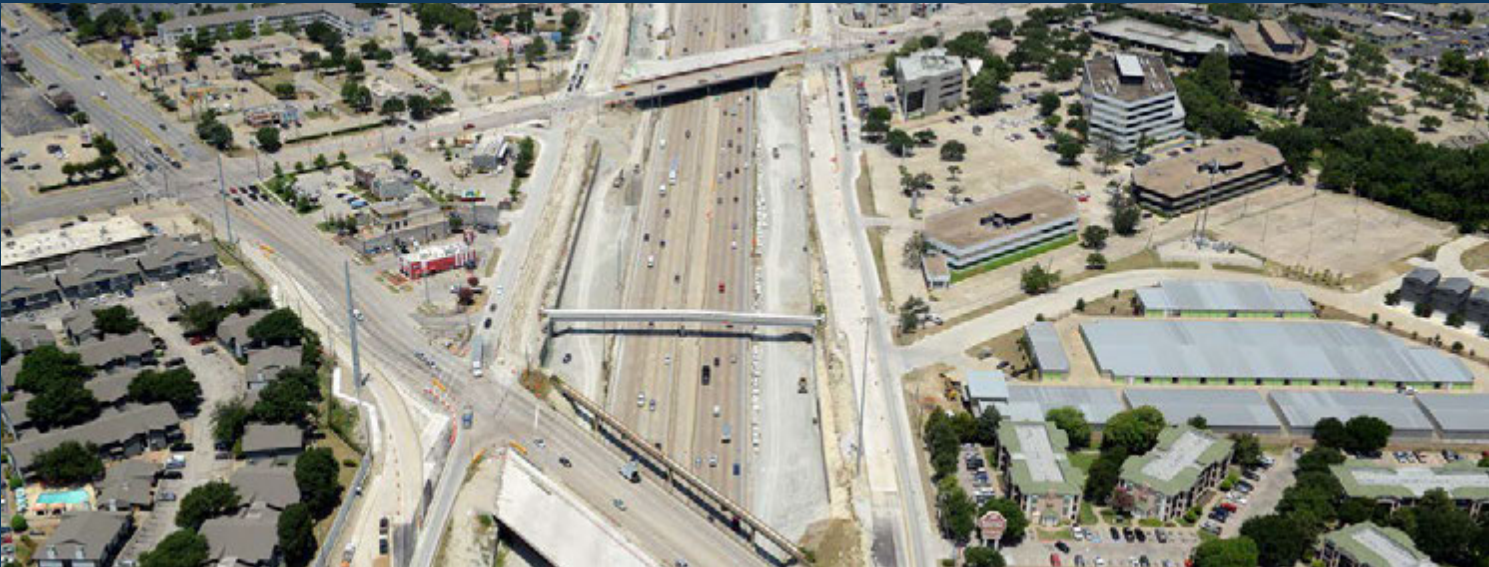
Abrams Road and Forest Lane new bridge sections await lane striping to accommodate traffic through the intersections.
