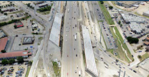
Beams set for the new I-635 frontage road bridges at Northwest Highway.
