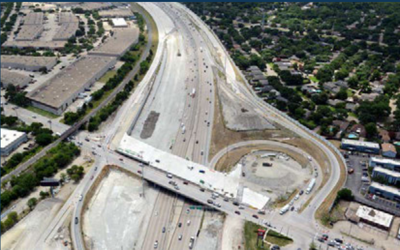
Royal Lane/Miller Road is being prepped to switch existing traffic onto the bridge's newly built section.
