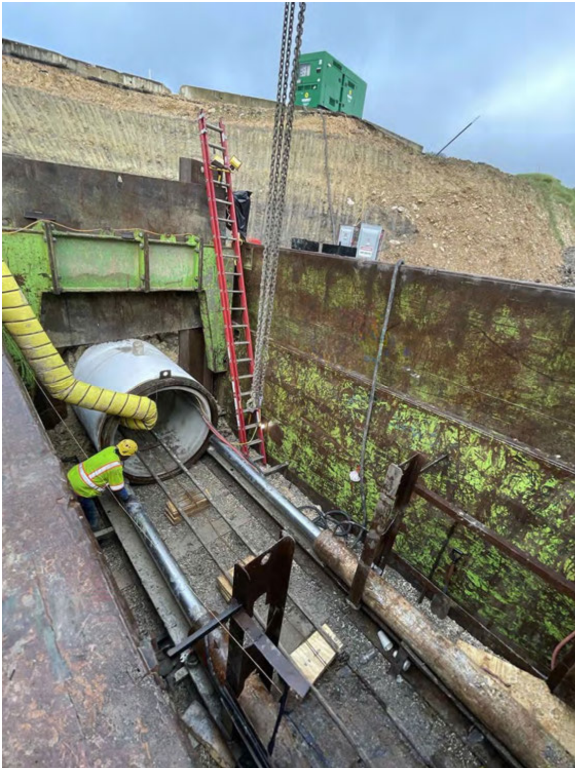
Boring a tunnel under Loop 1604 to expand drainage capacity.
