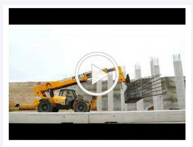
Work continues to progress on the I-35 NEX Central project in the area of Loop 1604 between Nacogdoches Road and Lookout Road. Crews continue to set drilled shaft cages, remove formwork extensions and pour concrete. The drilled shafts will carry columns up to 23 feet in height. Check out the latest video above to see all the work that is happening in this area.
