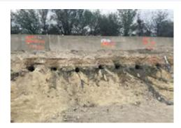
Crews have demolished existing retaining walls to make room for the drilled shafts work in the area of southbound I-35 and Judson Road. Drilled shafts and soil nail walls are used to give structural support to help stabilize the soil and prevent landslides.
