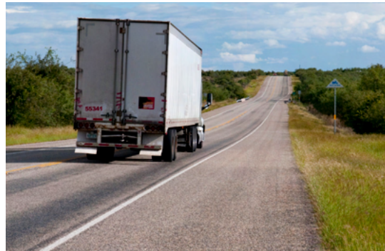
Figure 1. Typical seal coat application.
