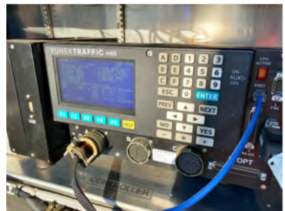
Front panel of controller in signal cabinet.
