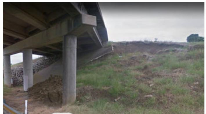
Shallow slope failure at the intersection of SE Loop 286 and Clarksville Street, Paris, Texas.
