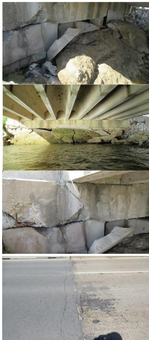
Figure 5. Structurally Deficient Bridge Components.
