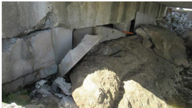
Figure 3. Deficiencies on the West Abutment of Bridge 101080069702030
