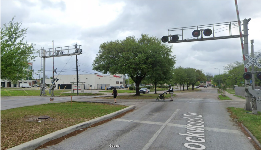
Figure 1: Grade Crossing at Lockwood Drive/UPRR Galveston Subdivision (Google Maps)
