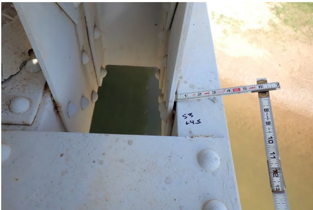
Pack rust with deformation at lower chord-gusset plate connection.
