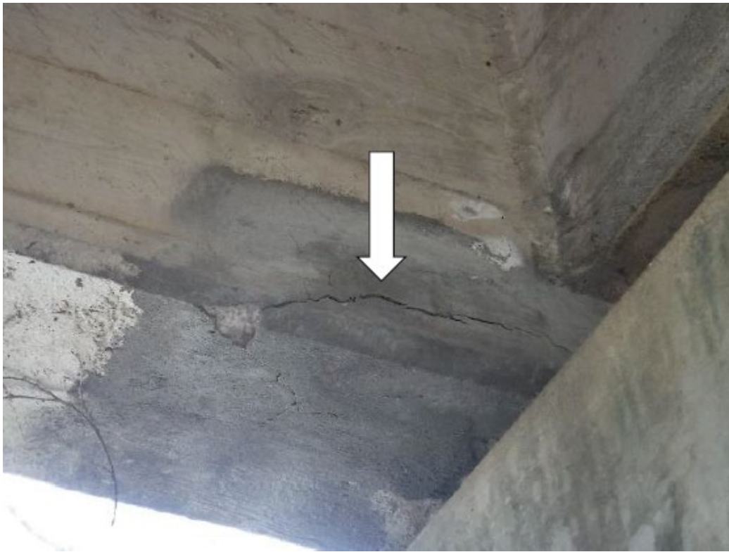
Delamination at girder stem
