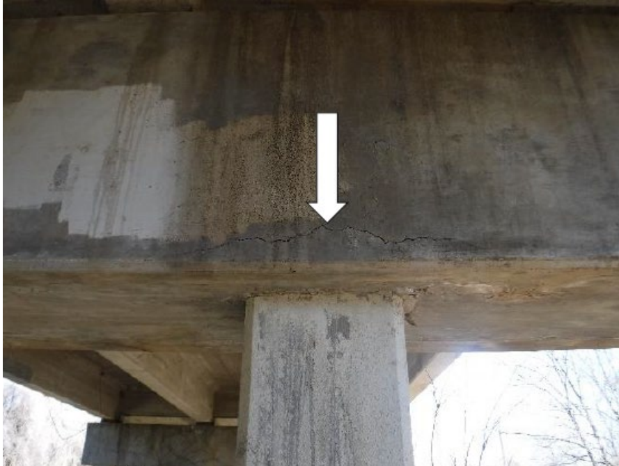
Delamination at substructure
