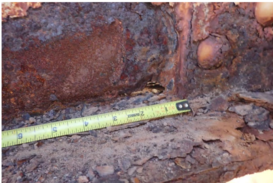
Corrosion at stringers
