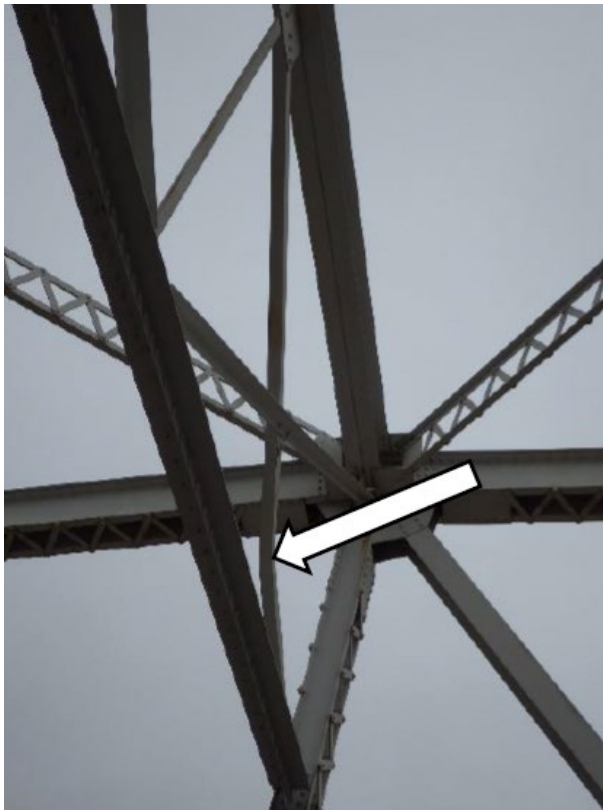
Distorted portal bracing member at location of previously repaired impact damage.
