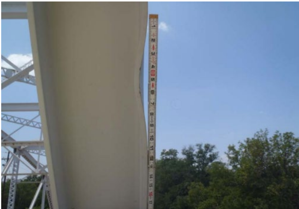
Impact damage to end post
