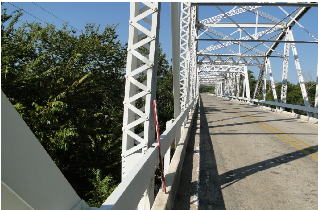
Bent vertical member at location of previously repaired impact damage (U2-L2).
