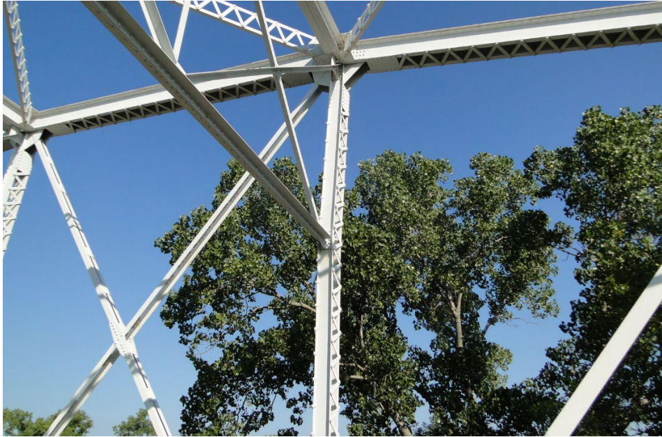
Bent vertical member at location of previously repaired impact damage (U3-L3).
