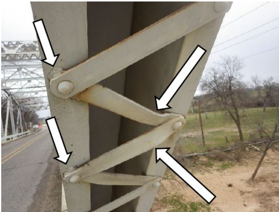
Distorted lacing and welded repair at location of previously repaired impact damage.
