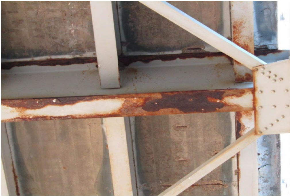
Typical floor system corrosion
